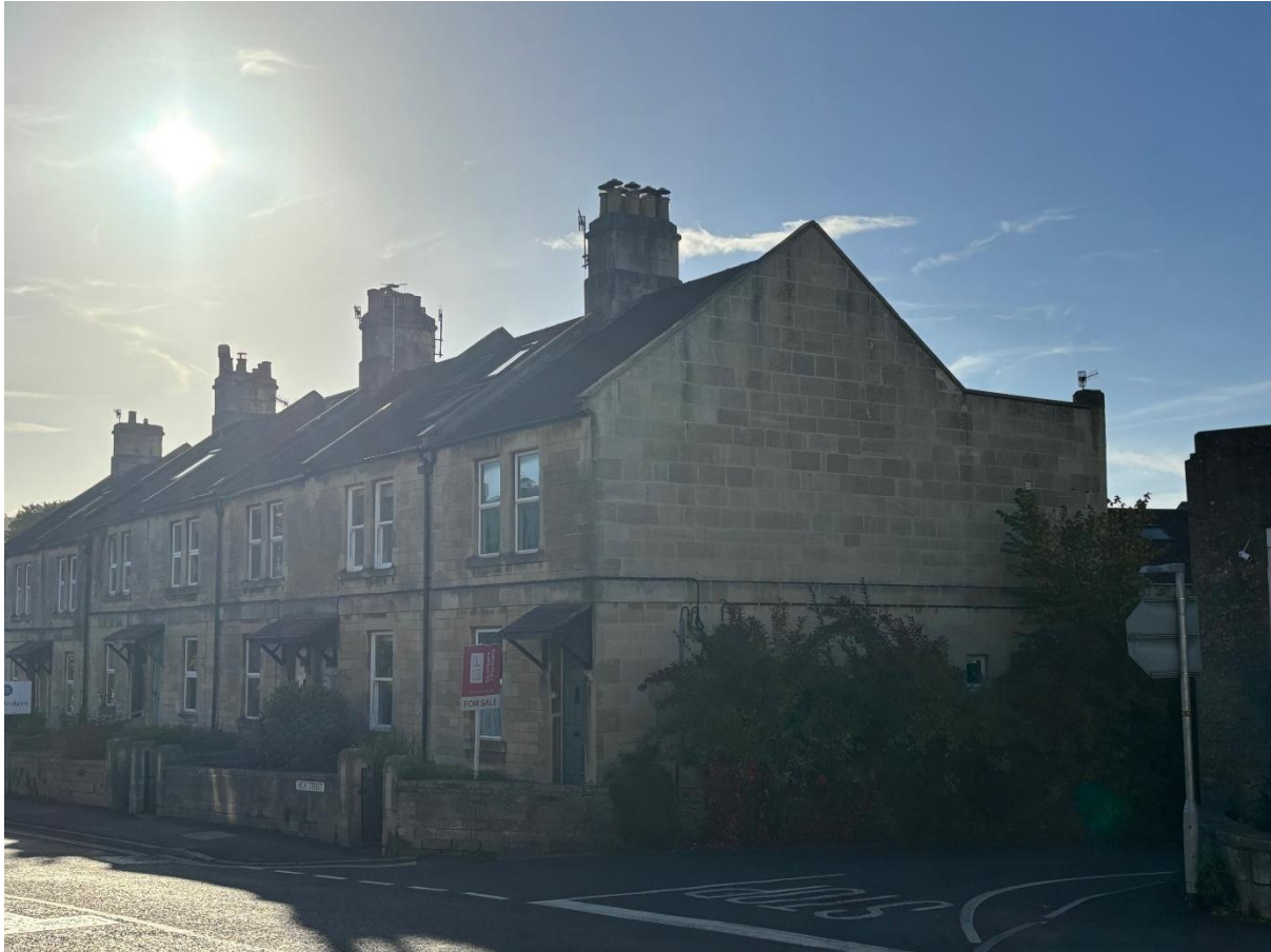
1 The High Street Box
