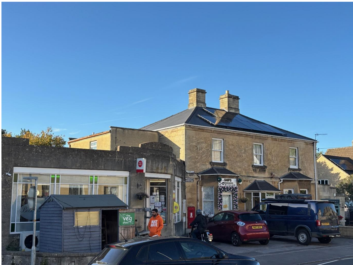
Post Office, opposite a Listed building with first floor extension
