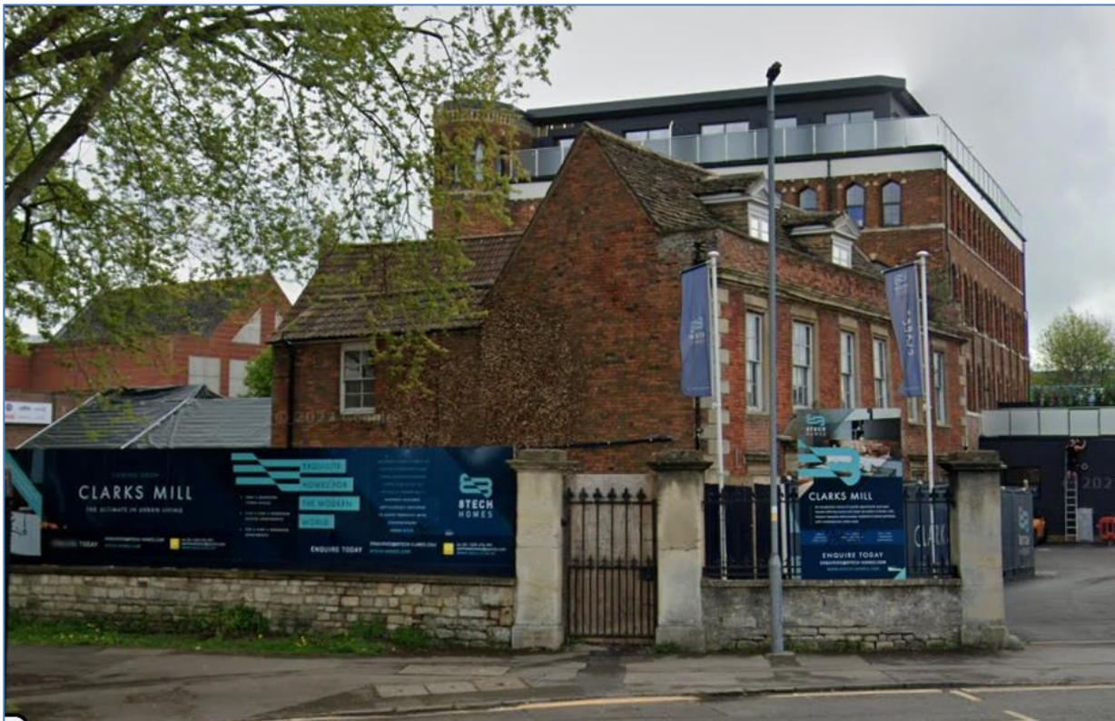
Figure 1 – Development Site (view from Stallard Street, extracted from Google Streetview, image captured May 2023).
