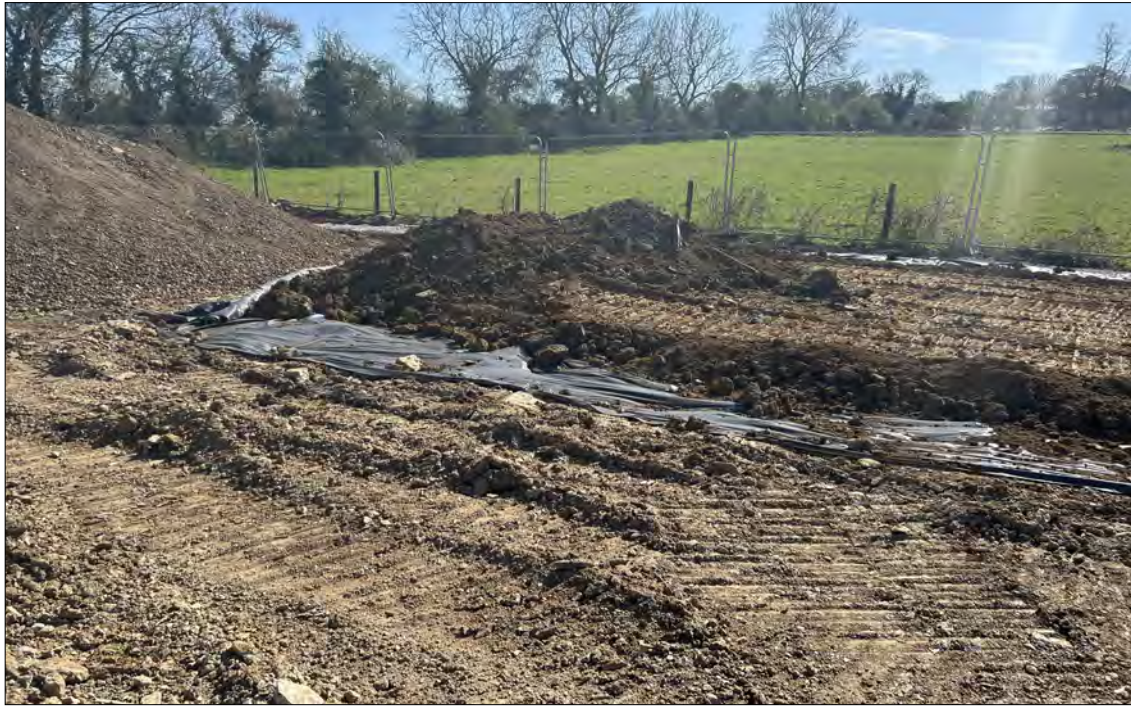
Laying of membrane and sub-base material
