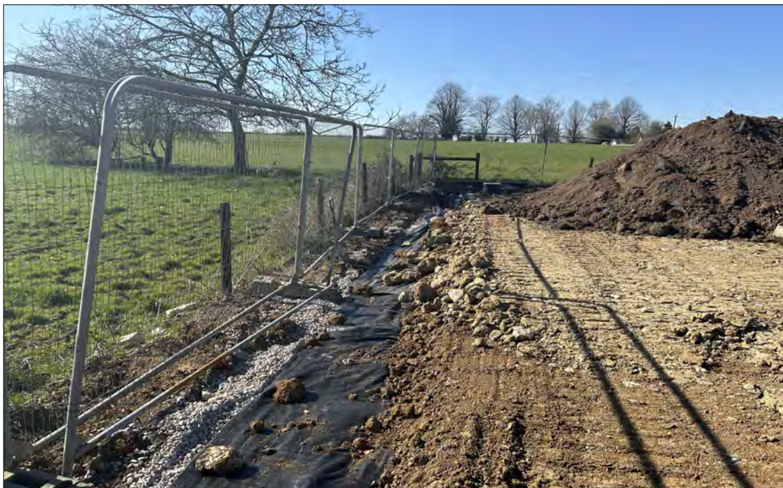
Laying of membrane and sub-base material with stockpiled topsoil
