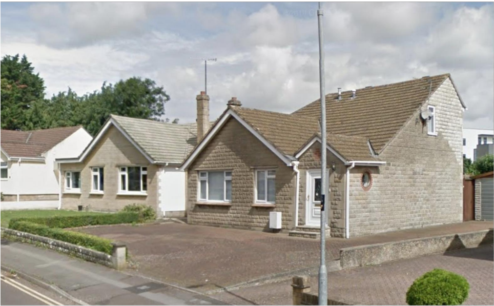
9 Sadlers Mead as viewed from front illustrating earlier 2 storey extension on rear
