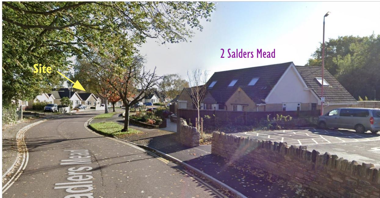
2 Sadlers Mead, attic conversion, as viewed from west looking to east
