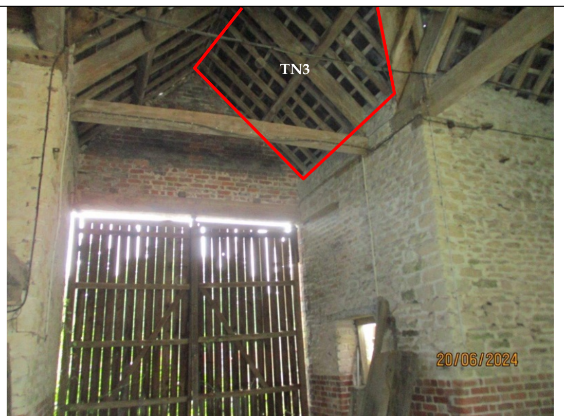
Figure 7c. Interior of barn B4 showing soprano pipistrelle roost feature (TN3) at southwest side
