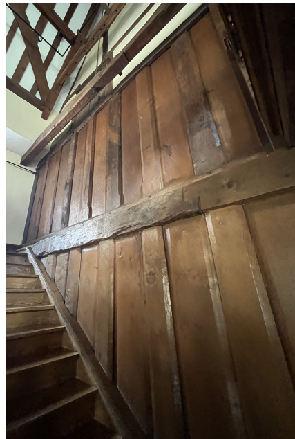
Example of existing Plank and Muntin wall to be replicated for new partitions
