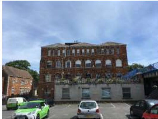
Photo 2: South west elevation
