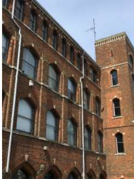
Photo 4: View of tower and north east elevation
