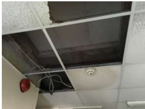
Photo 6: Internal view on top floor
