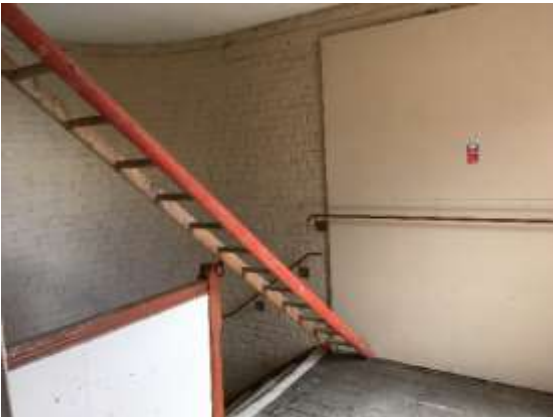
Photo 5: Internal view of tower
