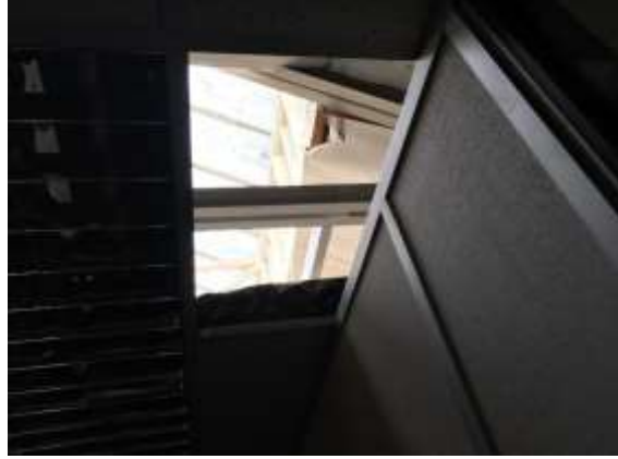
Photo 14: Internal view of glass roof
