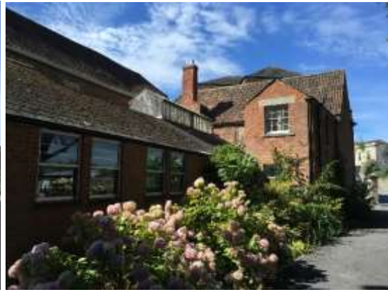
Photo 8: North east / north west elevation
