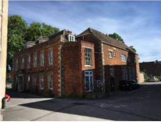
Photo 7: South view of building
