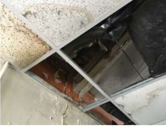
Photo 13: Internal view of single storey
