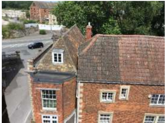
Photo 10: View of roof top on south east
