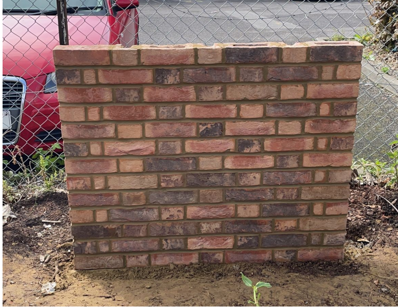
Sample panel of walling – Flemish bond style brickwork
