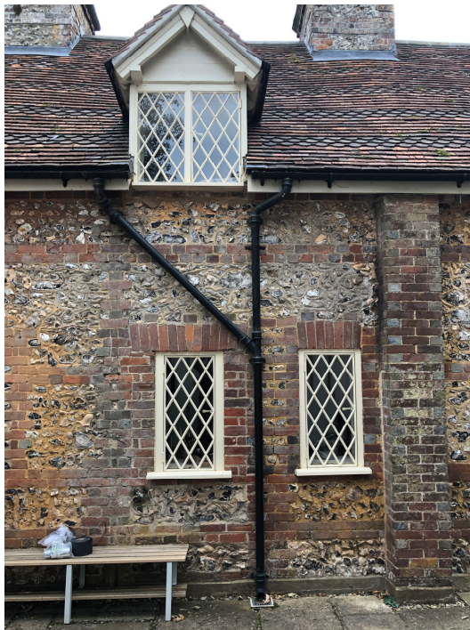
Former infilled doorway on north elevation
