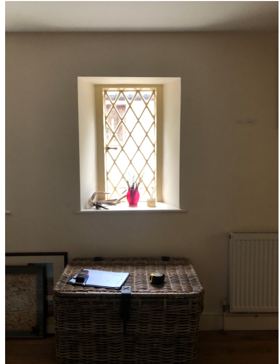
Internal photo of window to be removed
