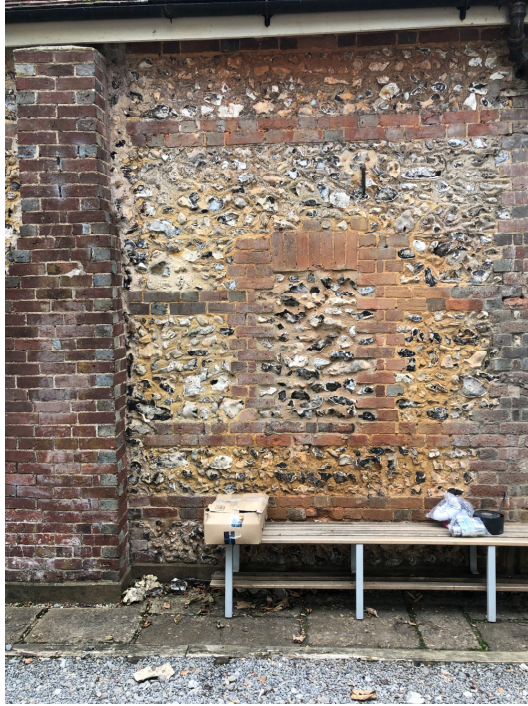
Former infilled window on north elevation
