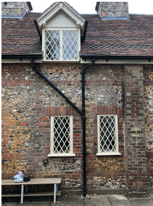
Former infilled doorway on north elevation
