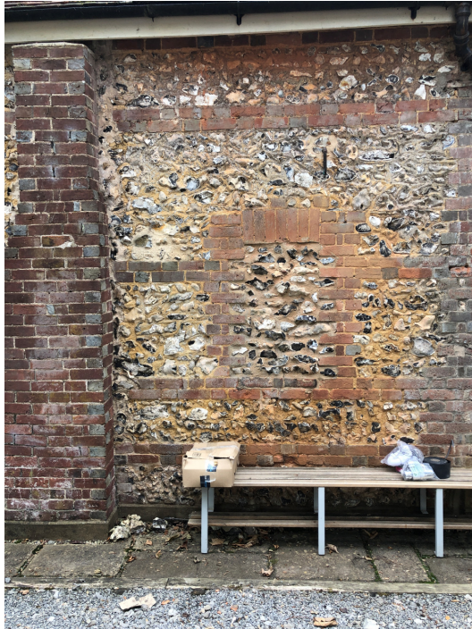
Former infilled window on north elevation
