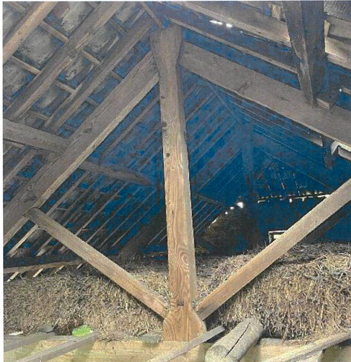
5. Typical King Post Truss
