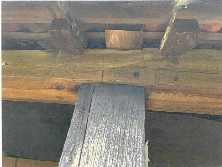
7. Eaves Beam Scarf Joint
