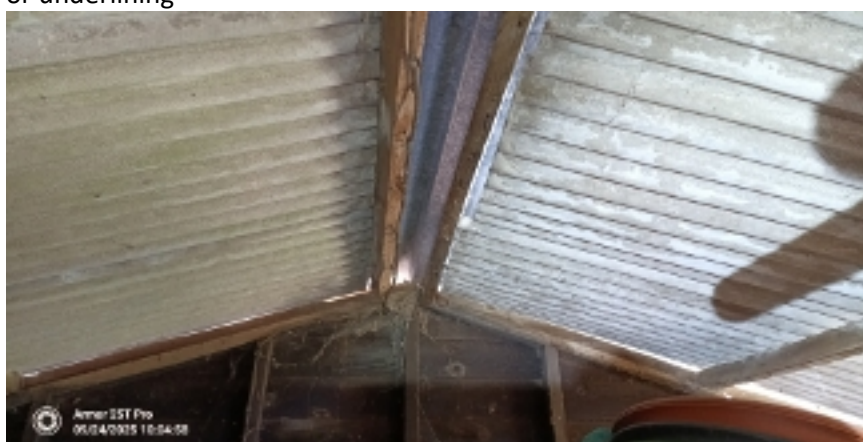
Photo 14. Internal corrugated asbestos type material roof with no cavity or underlining
