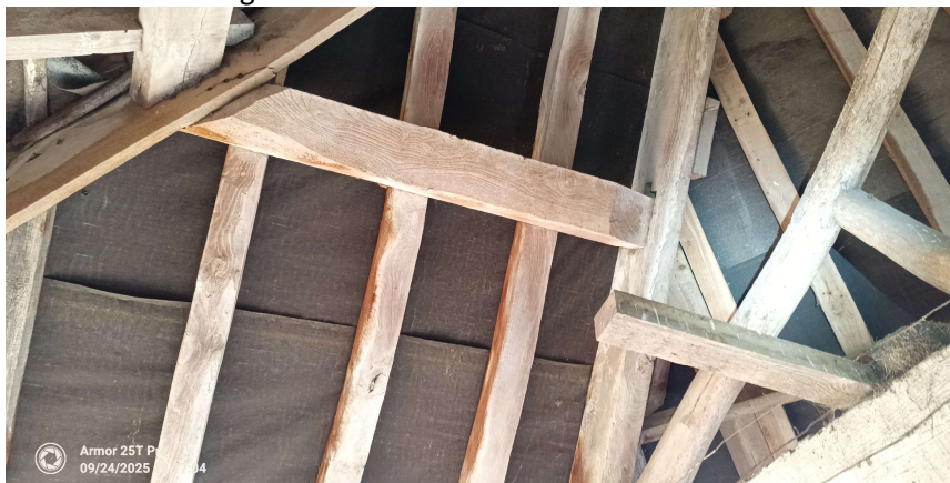
Photo 19. Showing some roof tiles underlined with felt
