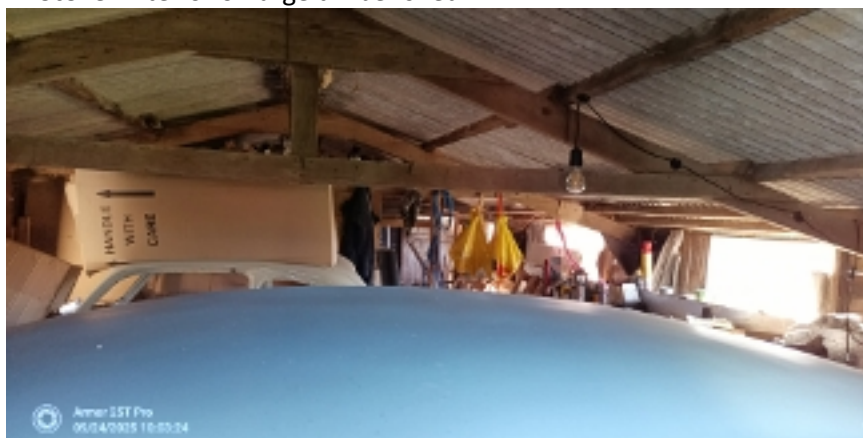
Photo13. Interior of large timber shed
