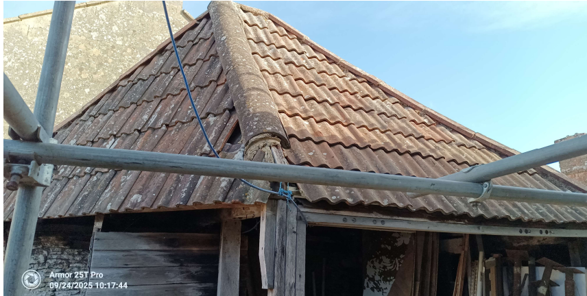
Photo 19. Showing some roof tiles underlined with felt
