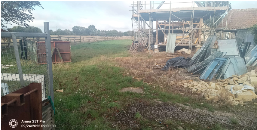
Photo 5. Looking north-west with the Cart Shed to the left, the large timber shed in the centre and part the Old Granary to the right
