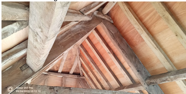
Photo 16. Showing open unlined sides of building
