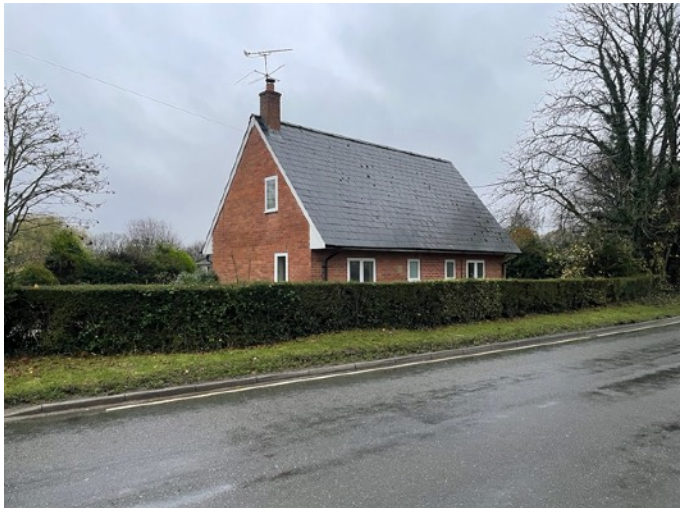
Ashley Cottage, South of the site
