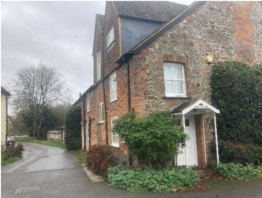
View of Ivy House from the Square, looking along South Street towards the boundary wall where the entrance gates would be introduced.
