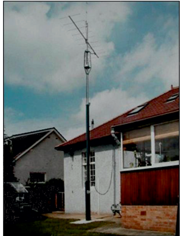
typical Amateur mast and antenna
