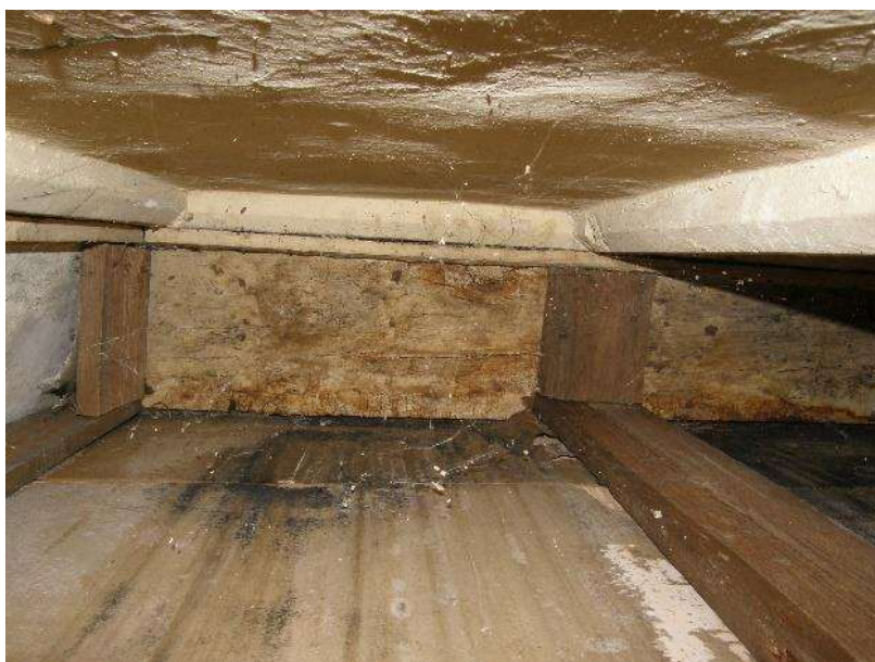
Fig.40 Interior of window void showing chamfered side of mullioned frame
