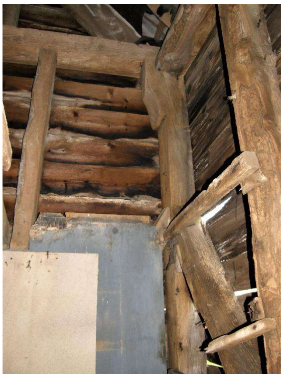
Fig.62 Former position of ladder to loft over
