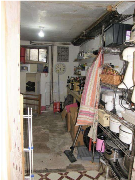
Fig.32 Chamfered beam in larder
