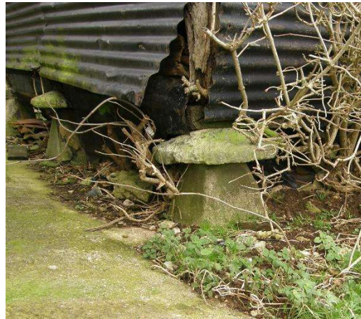
Fig.55 Sunk staddle in south-west corner
