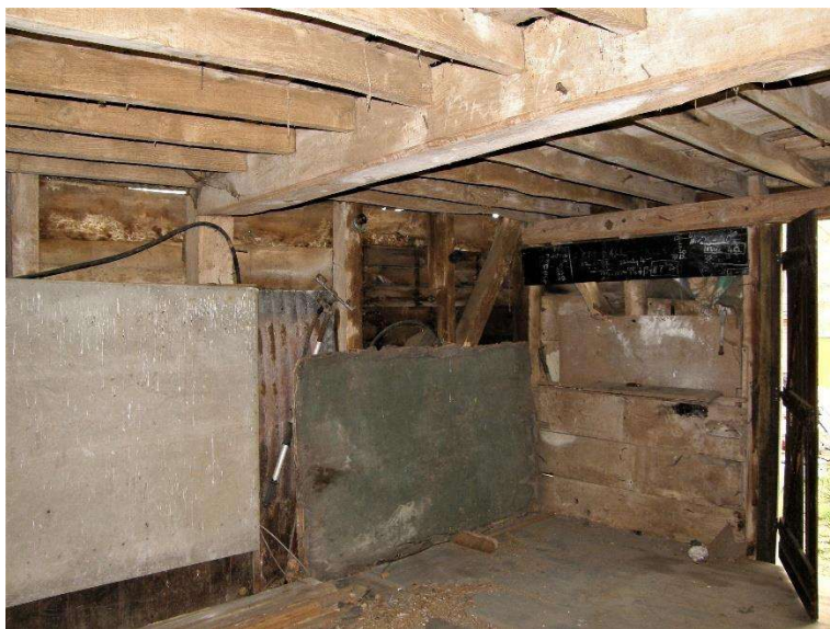
Fig.60 Interior with some remaining boarding on east wall
