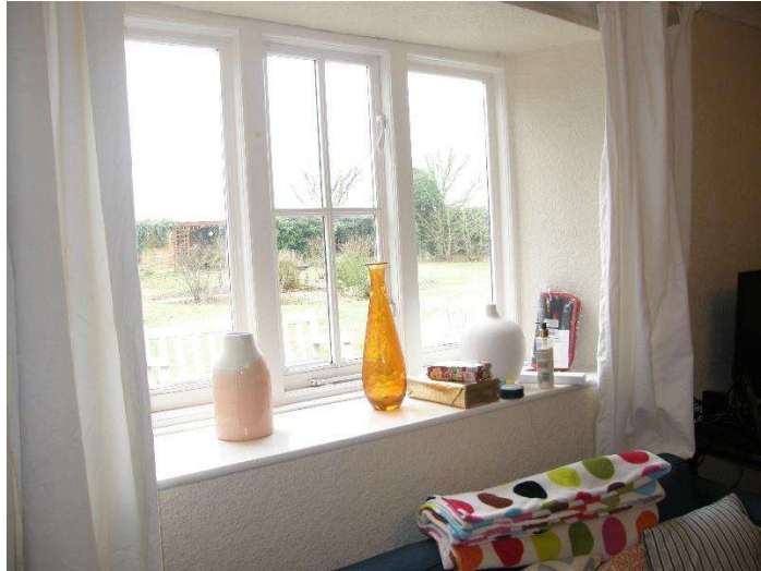
Fig.29 Old kitchen/sitting room window
