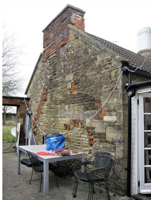
Fig.19 South gable end of kitchen
