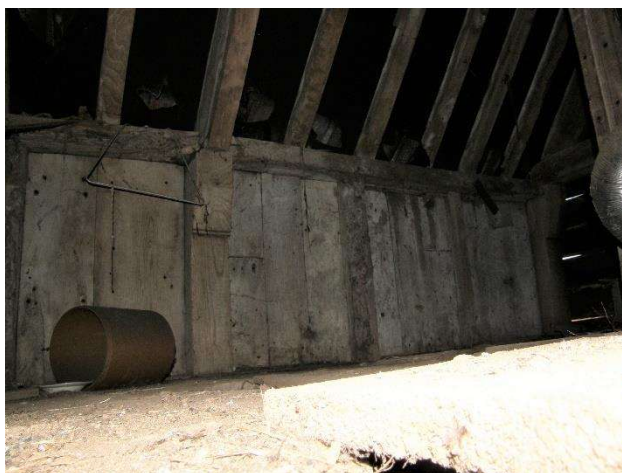
Fig.63 Vertical board lining in loft
