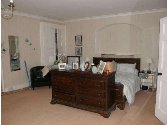
Fig.41 Possible blocked window on west wall
