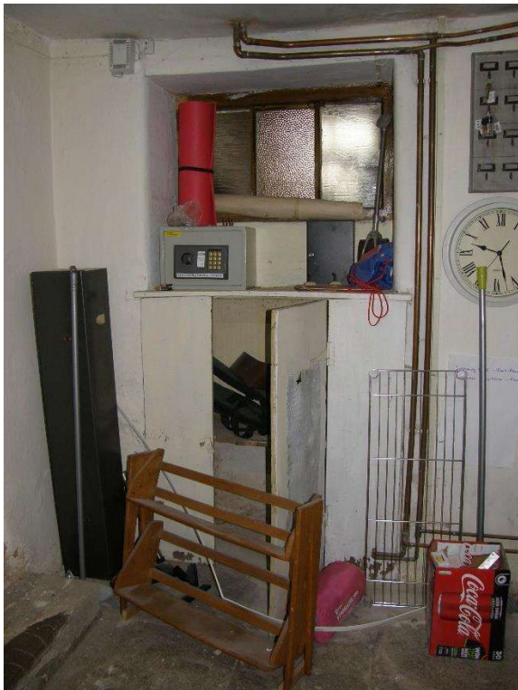
Fig.34 Former doorway from larder to front range
