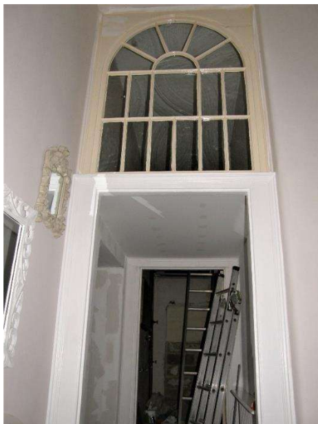
Fig.43 Borrowed light to rear of first floor
