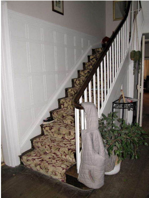
Fig.22 Straight flight stair
