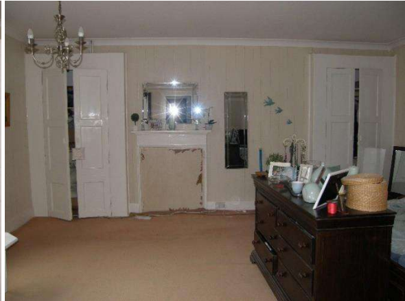
Fig.42 Blocked fireplace and built-in cupboards
