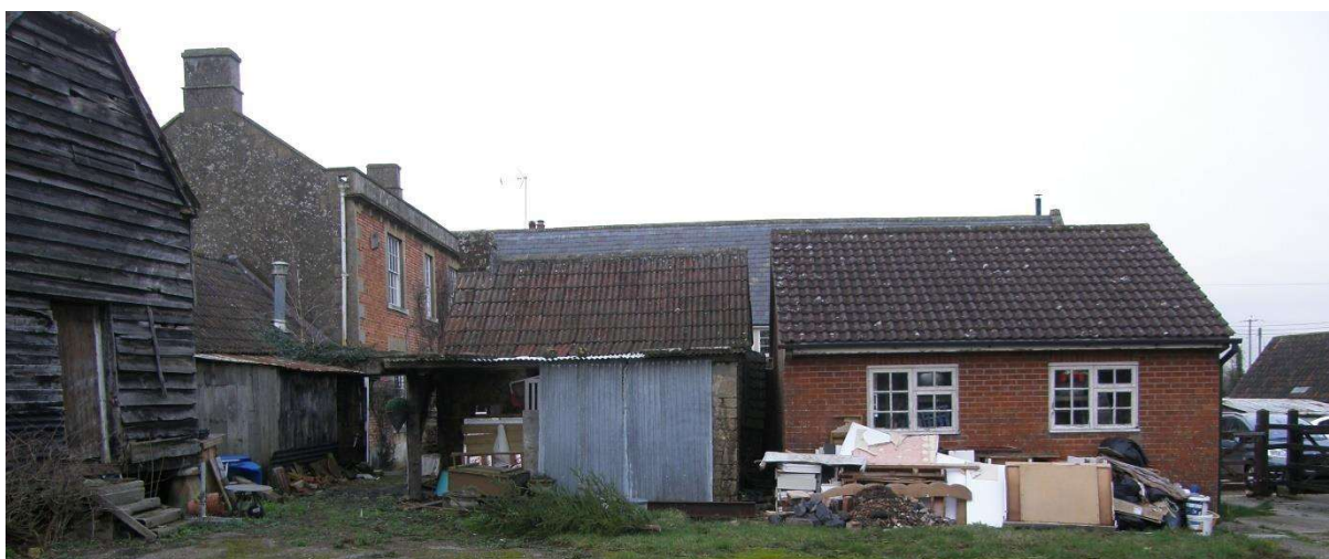
Fig.64 Rear of wash house and brick building replacing two stone pigsties with yards
