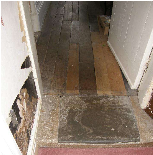
Fig.23 Limestone step with Pennant sandstone repair
