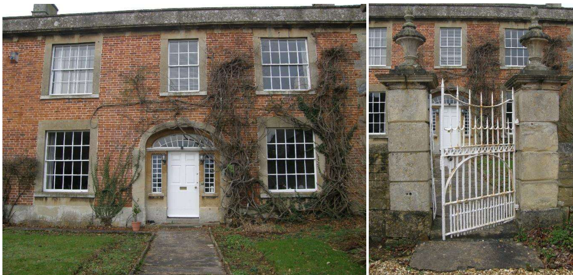
Fig.13 Main east elevation Fig.14 Rusticated gate piers with urn finials and probably original gate
