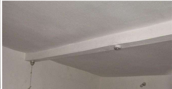
Fig.48 Plain beam dividing ceiling
