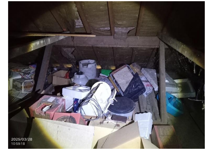
Photo 6: Internal loft void of B1.
