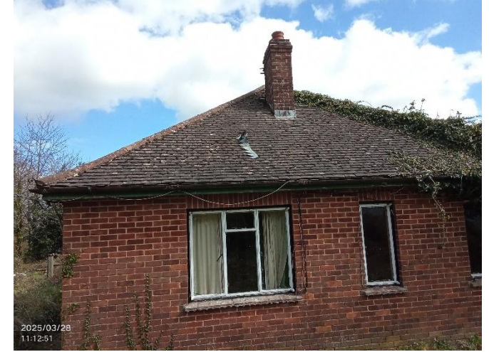
Photo 3: West view of B1.
