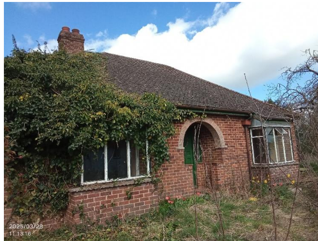
Photo 2: South view of B1.
