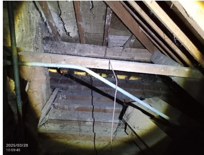
Photo 8: Internal loft void of B1.
