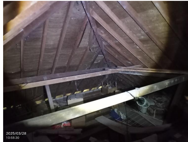
Photo 5: Internal loft void of B1.
