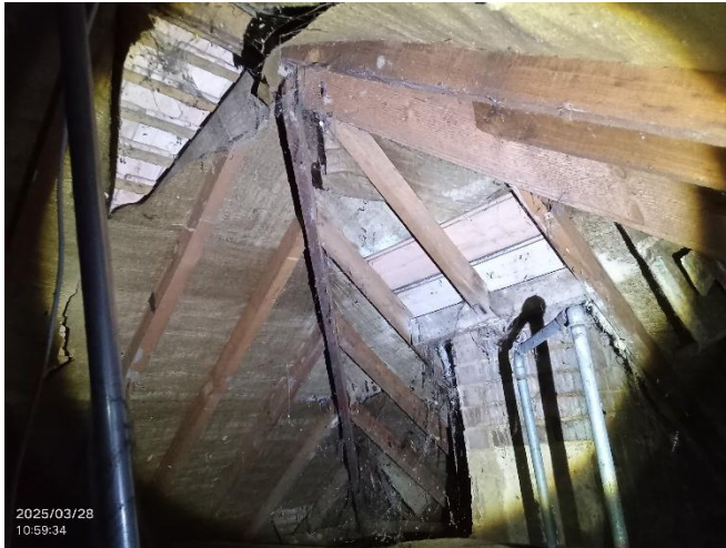
Photo 7: Internal loft void of B1.
