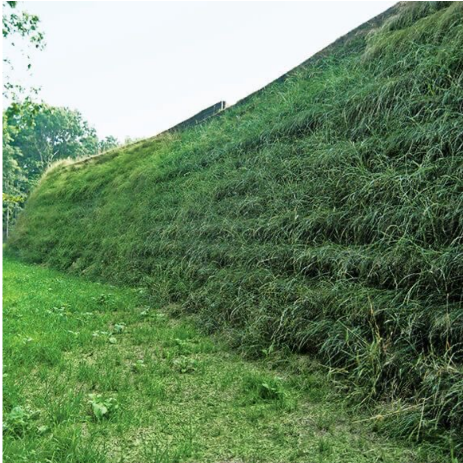
Example image of Gabion wall with plant plugs
