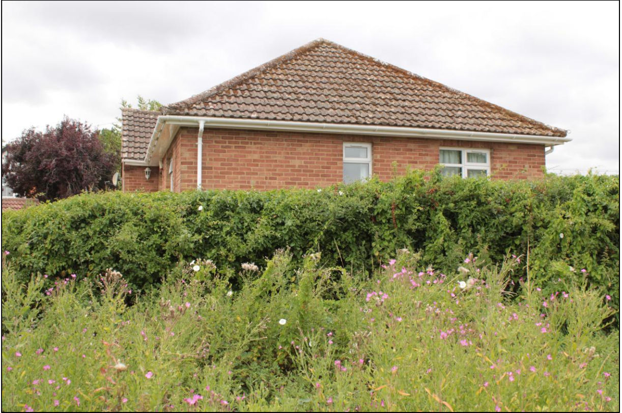
Photo 7 West facing view towards no. 82 High Street on higher ground.
