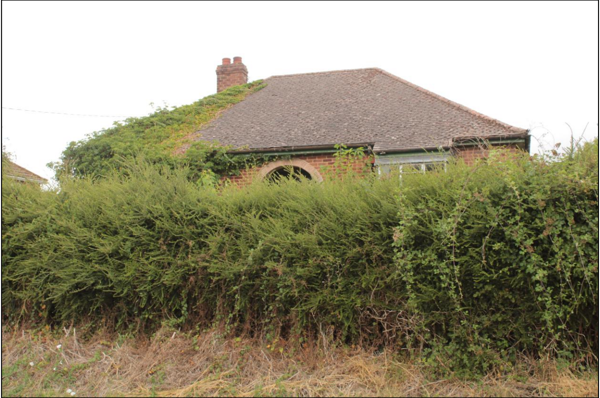
Photo 9 Northwest facing view of the Project Site from High Street, opposite the grade II listed 92 High Street. Views from the heritage assets opposite are curtailed by the rising north bank of the earlier sunken lane, which continues to rise to the rear of the modern 85 High Street. The same applies to public views from High Street, which are reduced due to the high bank and hedging.
