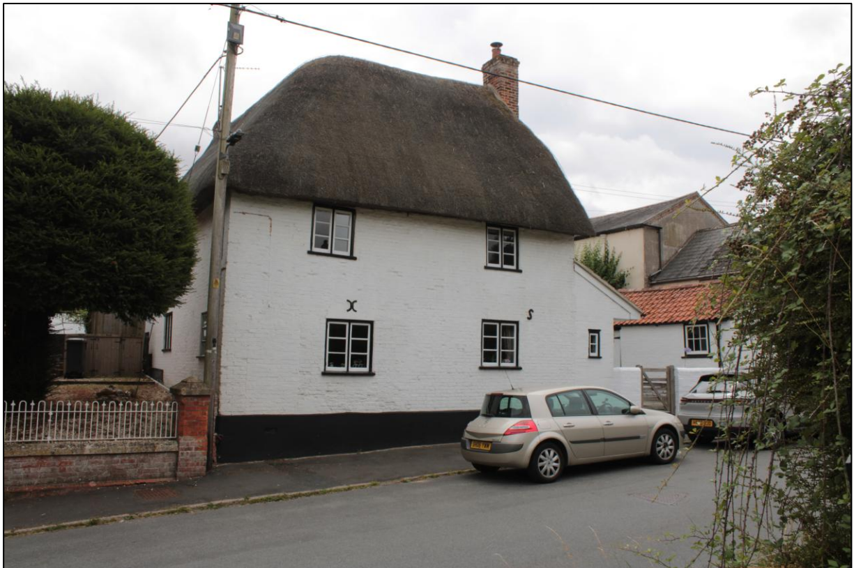
Photo 6 Northwest facing elevation of grade II listed no. 92 High Street, facing the Project Site.
