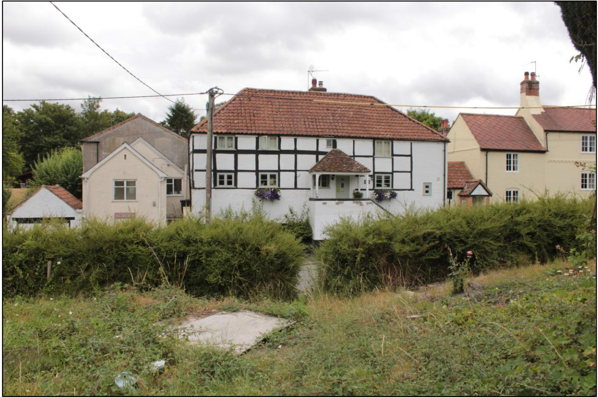
Photo 5 South facing view from the southwest end of the Project Site towards nos. 86 – 88 High Street.
