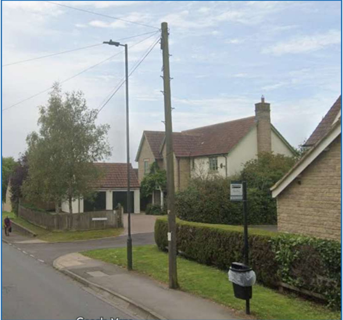
Figure 5 - Existing Lighting on Tetbury Hill (Google Maps, September 2023)
