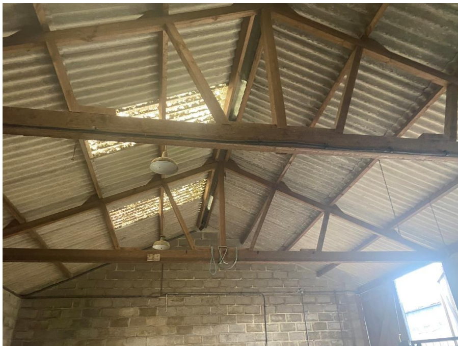
Plate 4: Interior view of main barn
