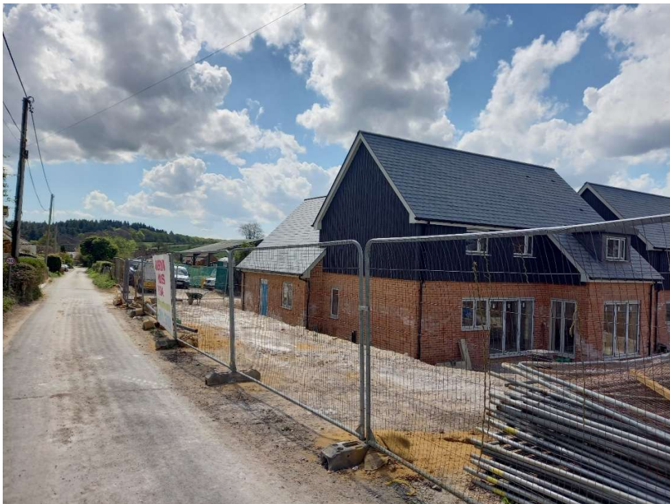
View looking down Witt Road with new dwellings set at lower level
