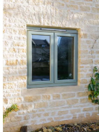
Flat arch built in random rubble
