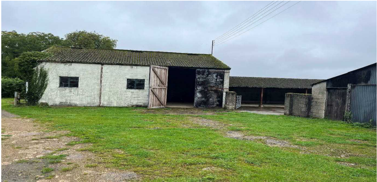
View of barn looking north at southern elevation RWPs
