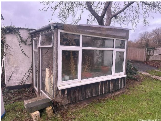
Photo 7: Conservatory on garage (B2).
