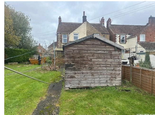
Photo 3: Shed (B1) in the south of the site.
