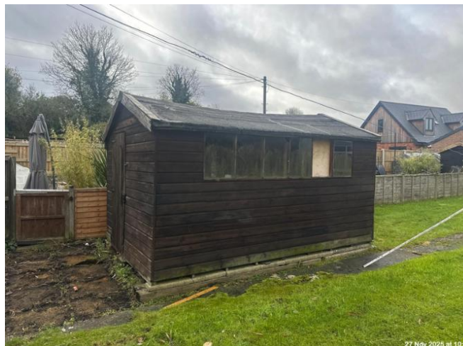
Photo 2: Shed (B1) in the south of the site.
