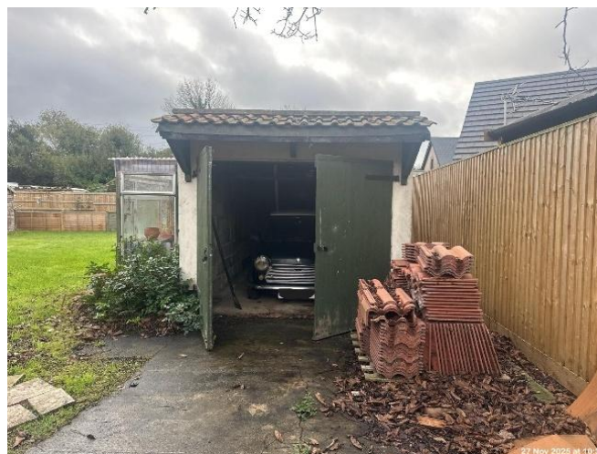
Photo 5: North elevation of garage (B2) in west of site.
