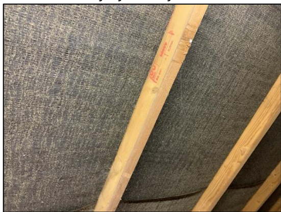
Photo 12 Internal roof of garage
