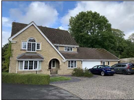
Photo 1 Front East elevation
