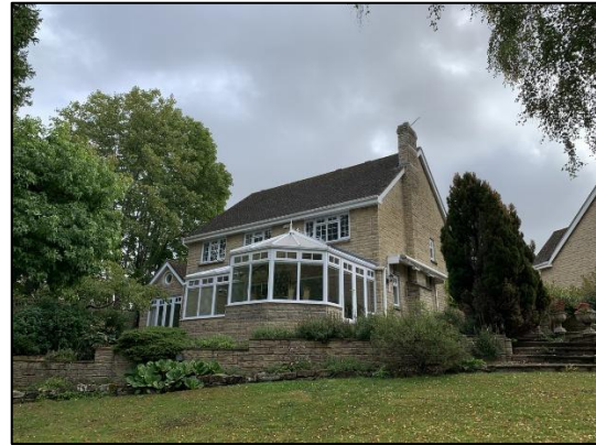
Photo 2 Rear West elevation
