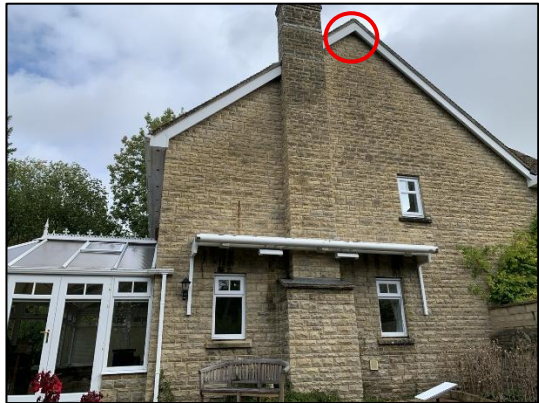
Photo 3 Side South elevation
