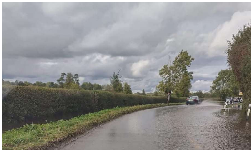
Fig 3.3.2 road outside entrance to Packhorse Corner, Nov 2024
