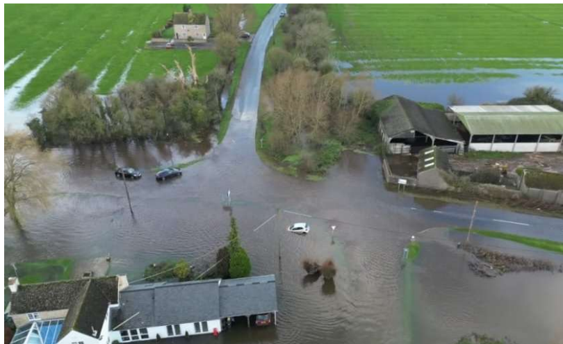
Fig 3.3.1 aerial photo of flooding, Nov 2024
