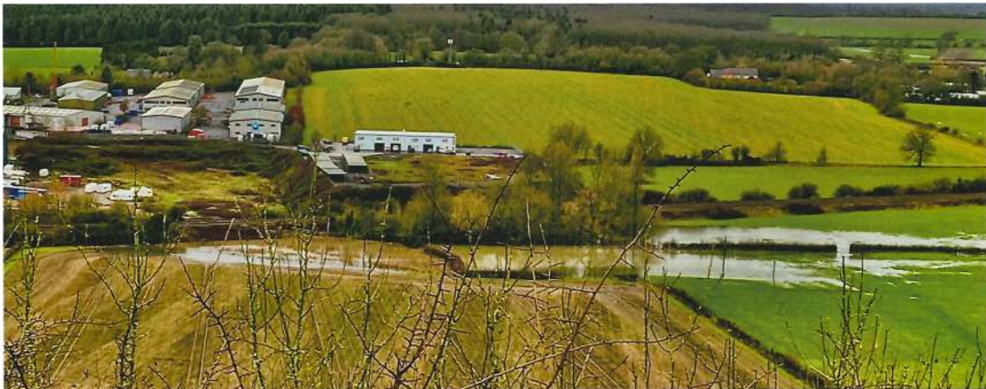
Figure 30: Floodwater ponding upstream of southern railway culvert in December 2023
