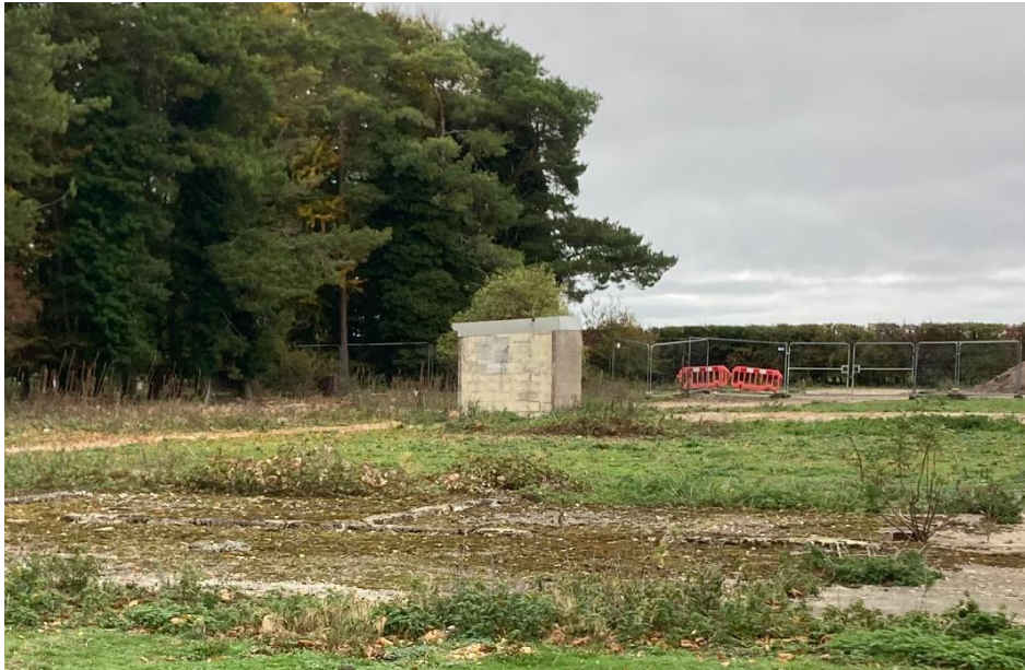
Figure 5. View of the small shed present on site (taken October 2025).
