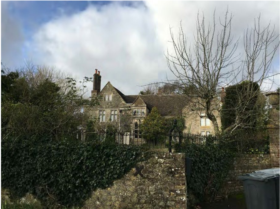
Plate 2: Parks Court viewed from the south.
