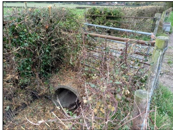
Photo 25: Culvert within the stream
