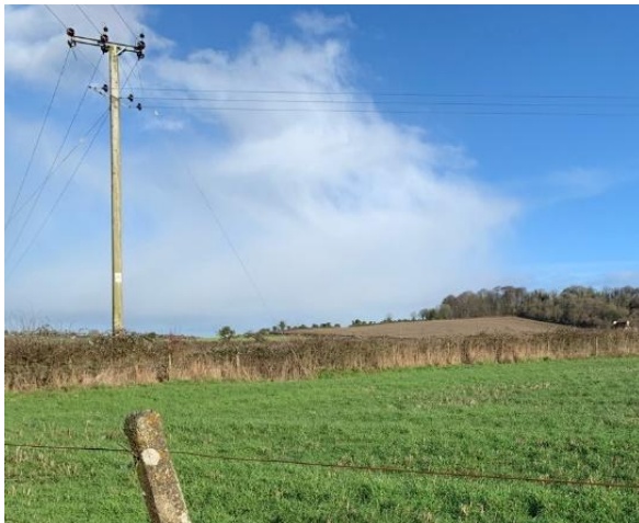
Photo 7 H2 from east
