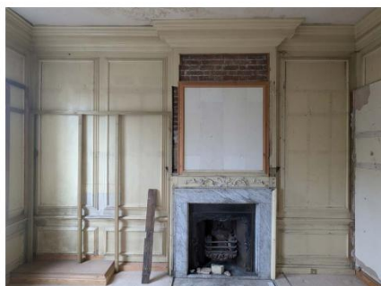
Existing condition: East wall
