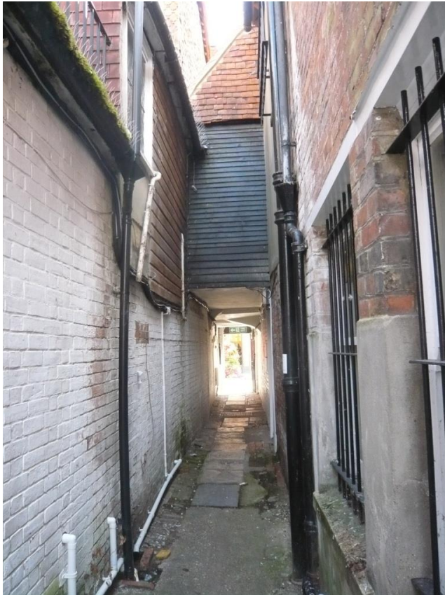
Fig.6 View from passageway looking towards High Street – two-storey gabled range with tile-hanging and timber cladding to left and single-storey flat-roofed structure beyond
