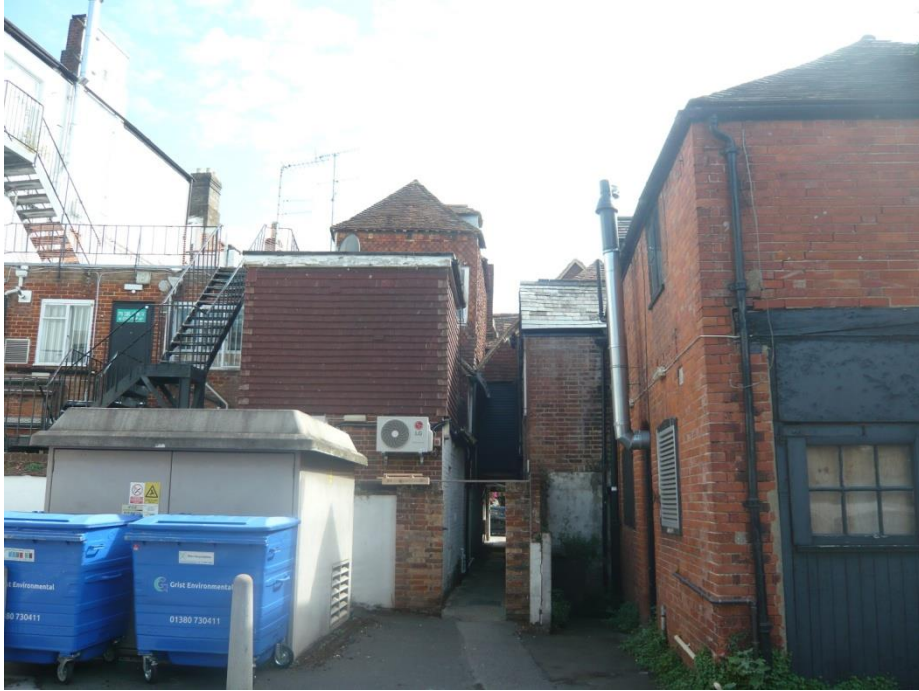
Fig.4 View of back of 10 High Street from rear service yard
