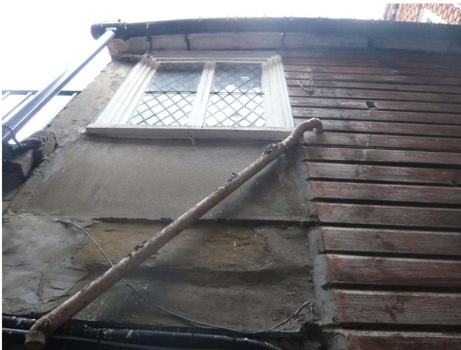
Fig.7 South side of two-storey gabled range with timber cladding
