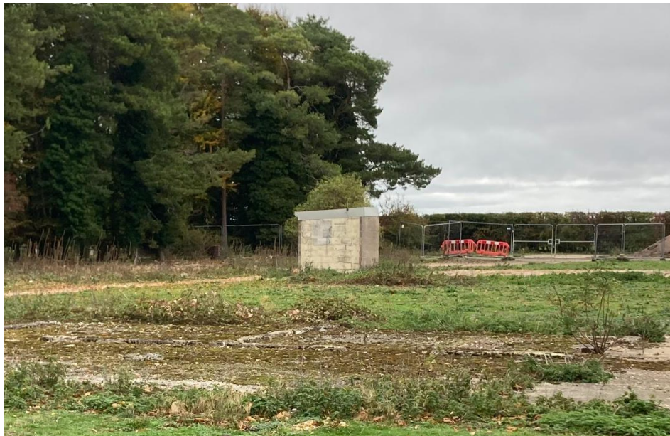
Figure 4. View of one of the buildings present on site (taken October 2025).
