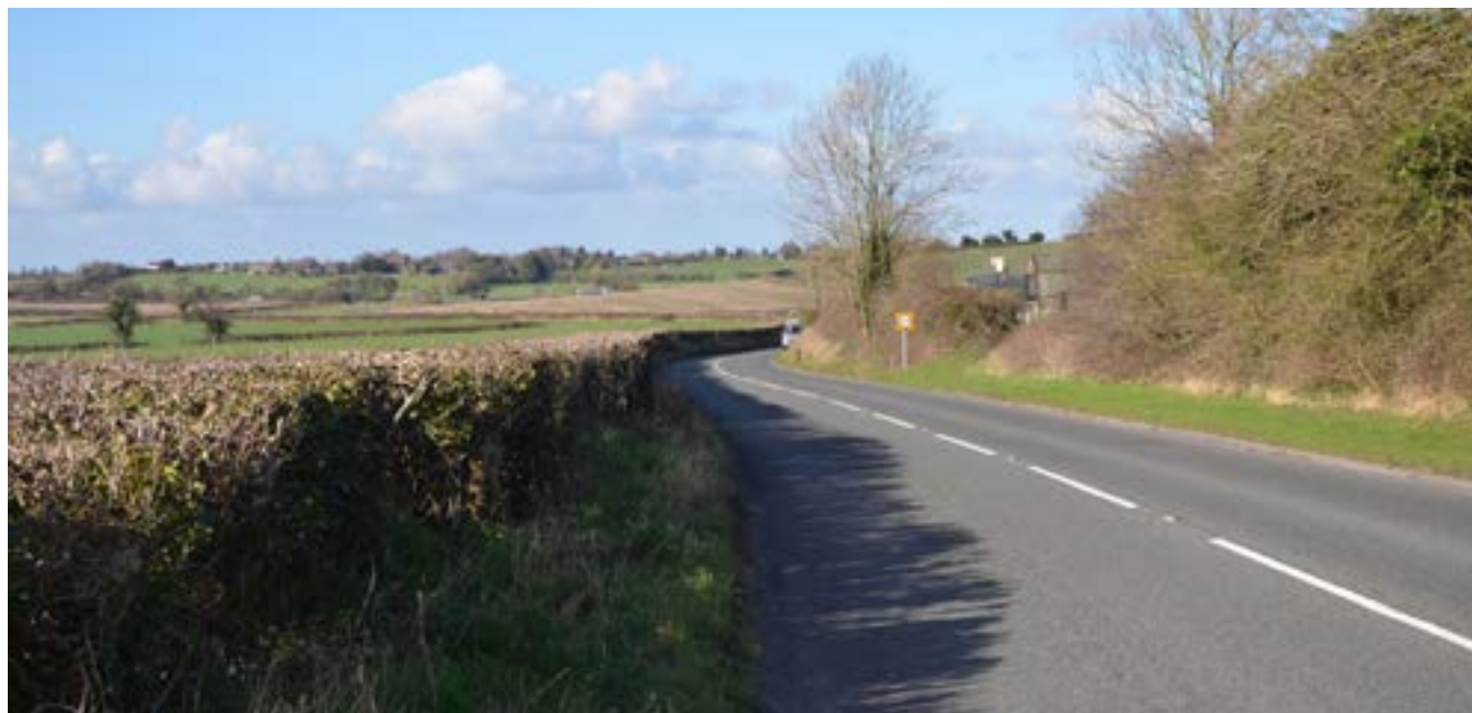
View along Westbury Road facing north
