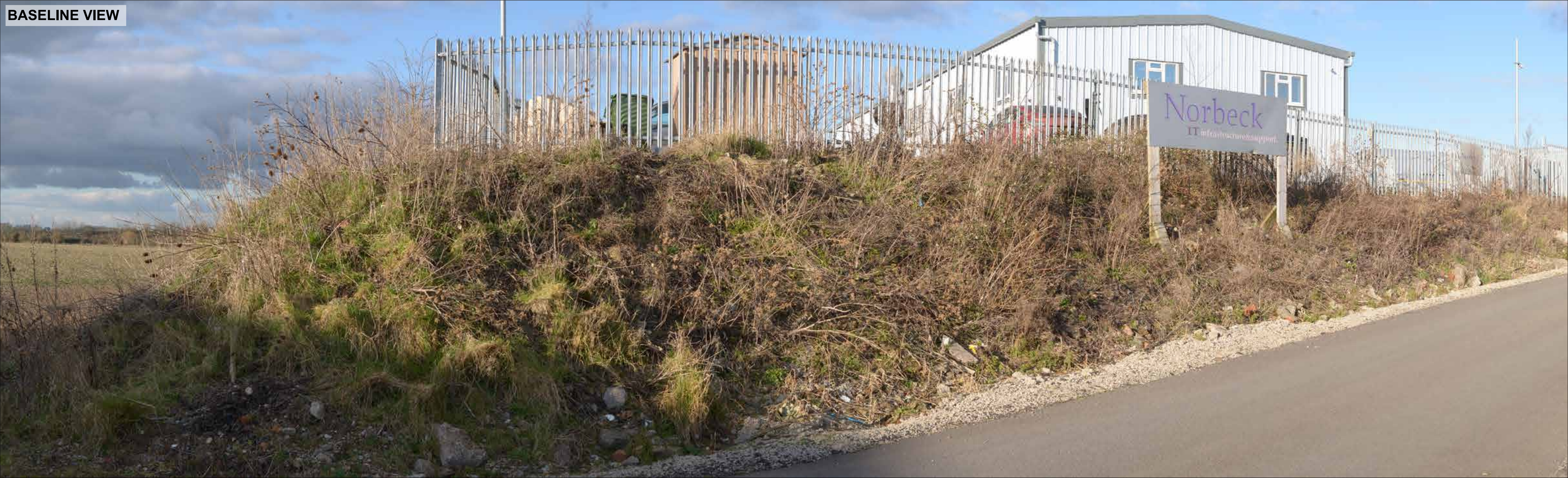
VIEWPOINT 17: VIEW FROM FURNAX LANE, LOOKING EAST TOWARDS THE SITE.
