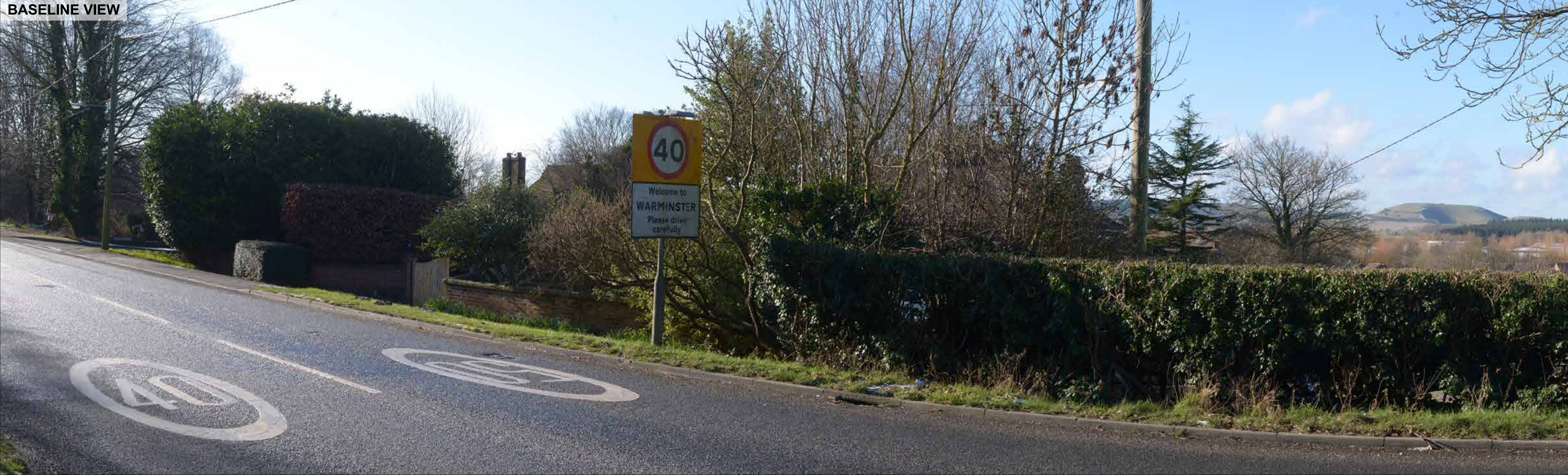
VIEWPOINT 01: VIEW FROM THE GRASS VERGE ALONG WESTBURY ROAD, LOOKING NORTH-EAST TOWARDS THE SITE.
