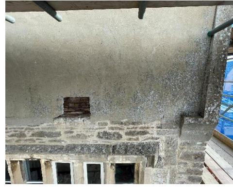
Close up images of Render(taken from scaffold erected for pointing repairs to stonework) - Image by Dolman
