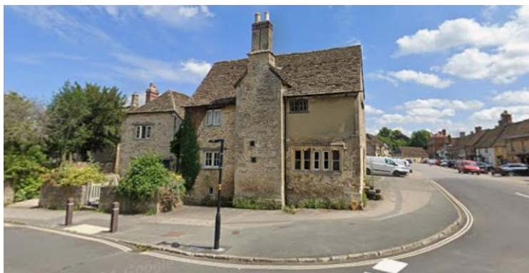
West Elevation of 15 High Street - Image from Google Street View https://www.google.com/maps/place/High+St,+Lacock,+Chippenham+SN15+2LQ/@51.4147709,-1.1231819
