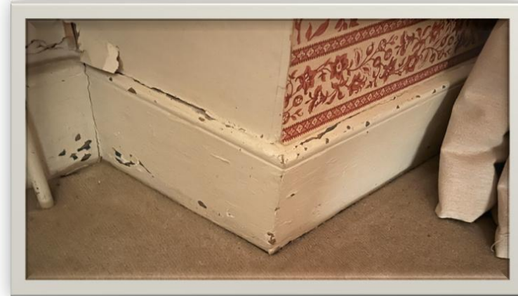
Timber Rotting due to moisture ingress
