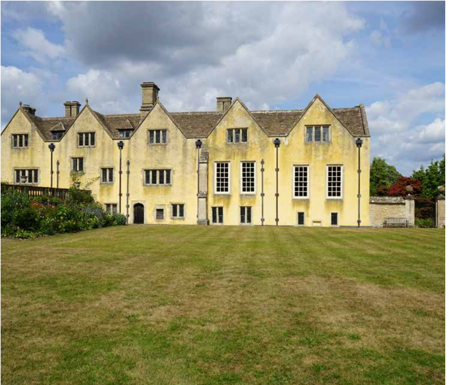
West elevation - pair of gables to the right 'original' and three gables to the left a c.1920 addition. The lawn in front is divided into two levels and separated by stone steps and a balustrade. This level difference accounts for the reduced height elevation to the north.
