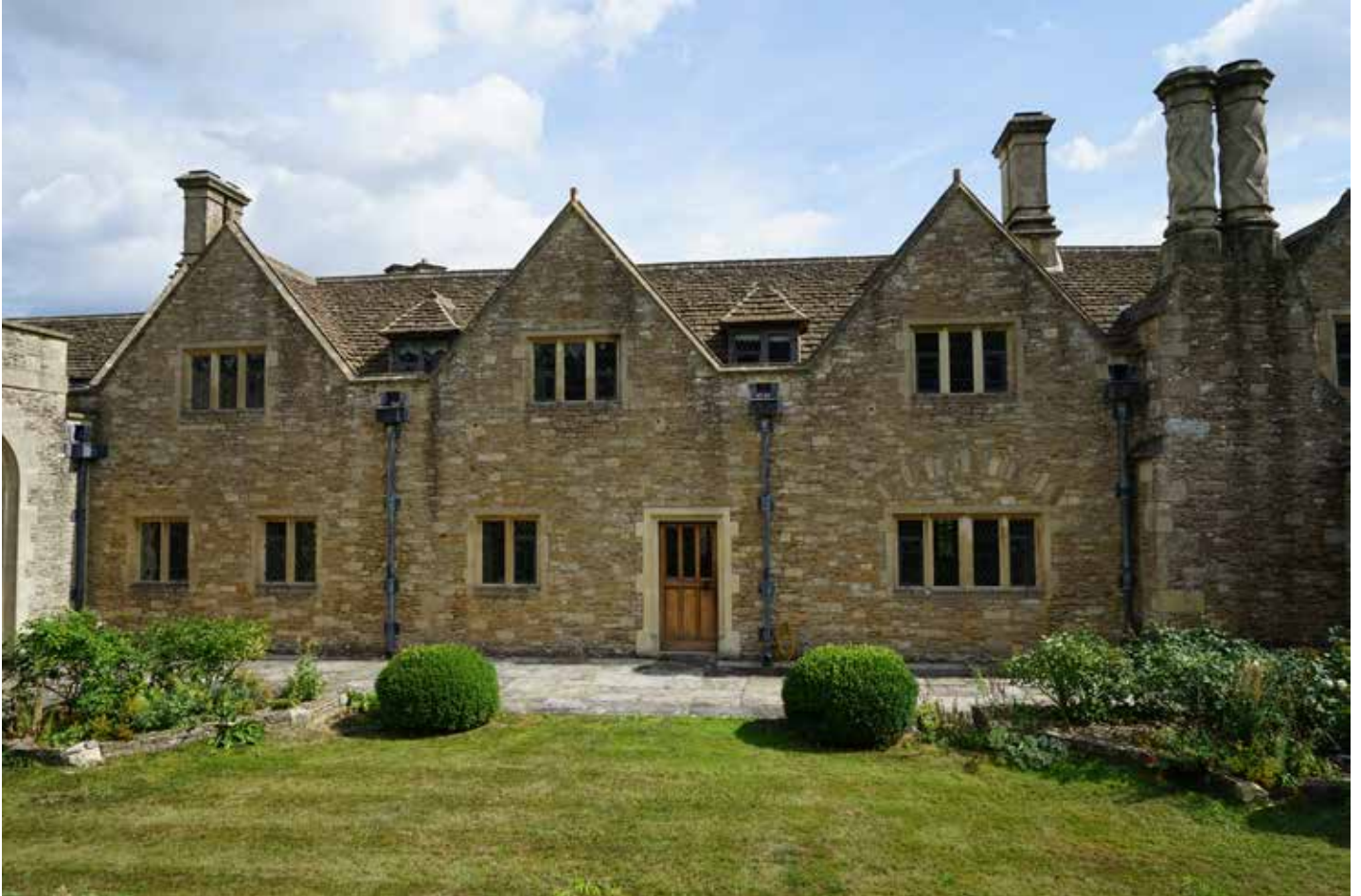
North elevation, 1920s construction and at first and attic floors levels only.
