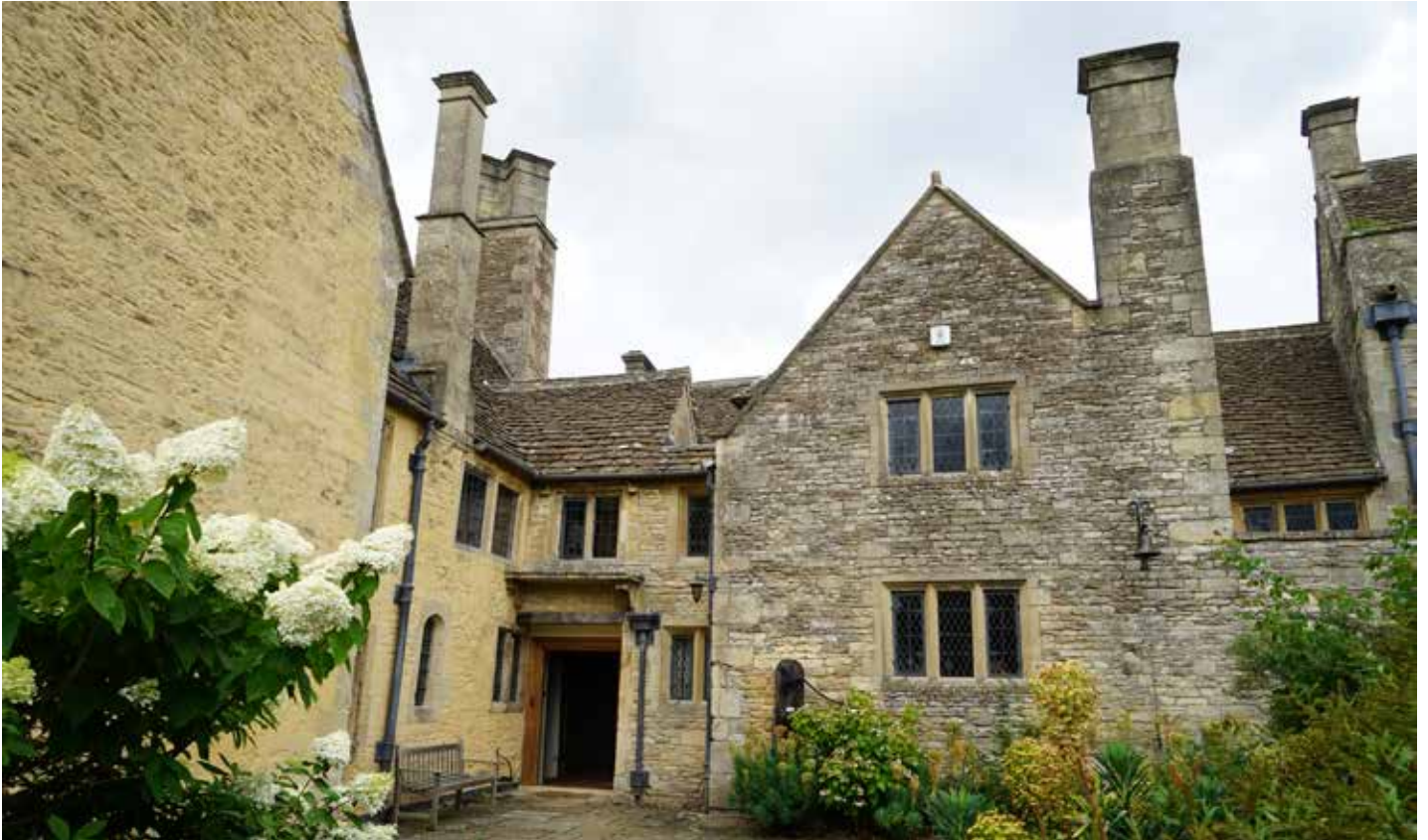
The short original range to the east of the main house, a with upper 2-light window and hoodmould over, and an open porch with long hood on carved 18th century brackets. To the right is c1920s service range added and linking to Dower House.
