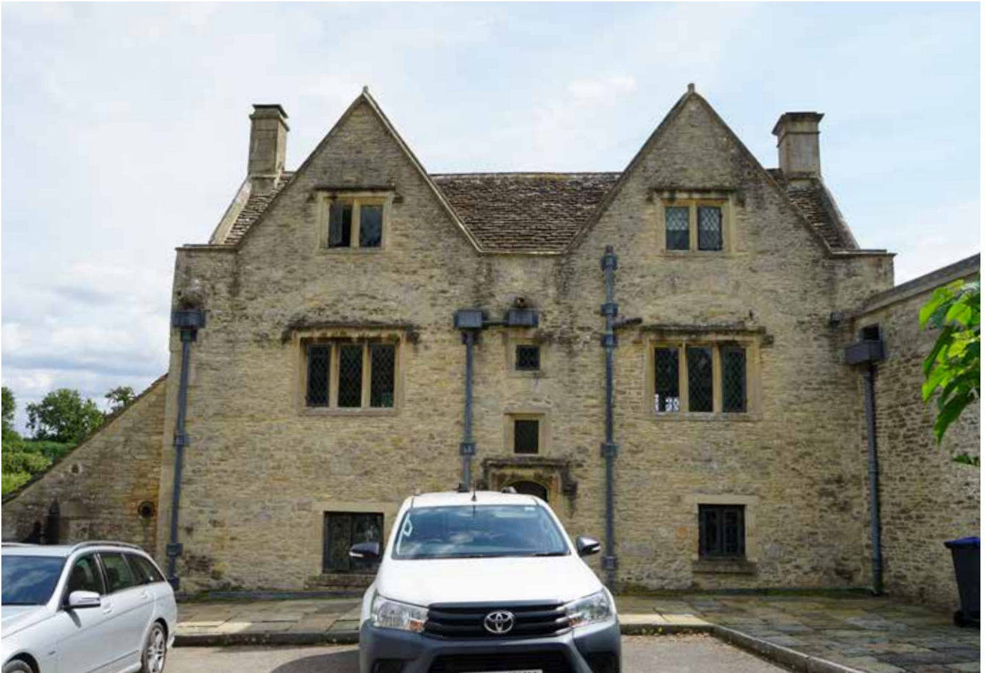
Dower House north elevation with central access door to half landing of stairs.
