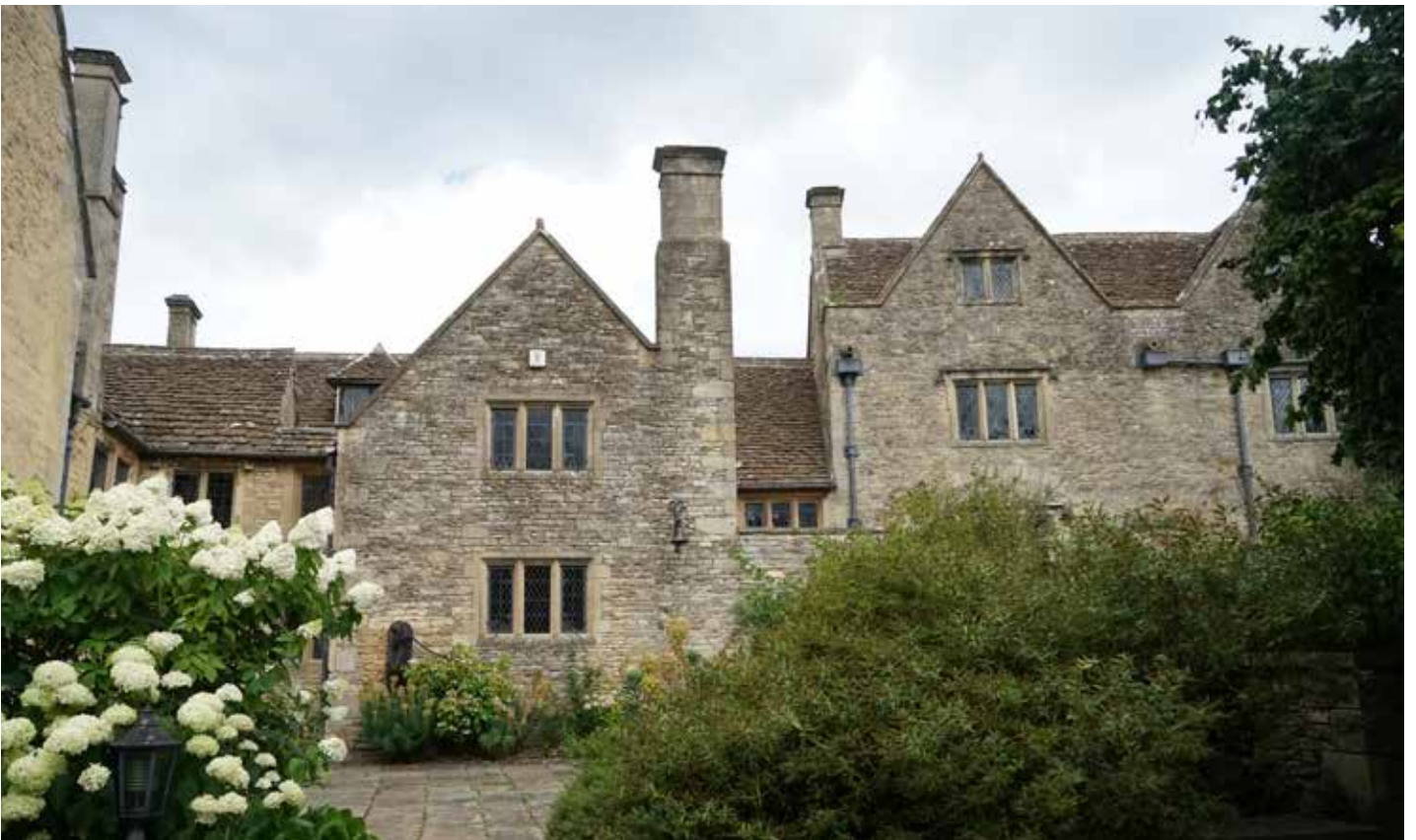
Linking early 20th century service range with three-light mullions lead light windows set centrally in gable and with corner chimney stack. Dower House to the right.
