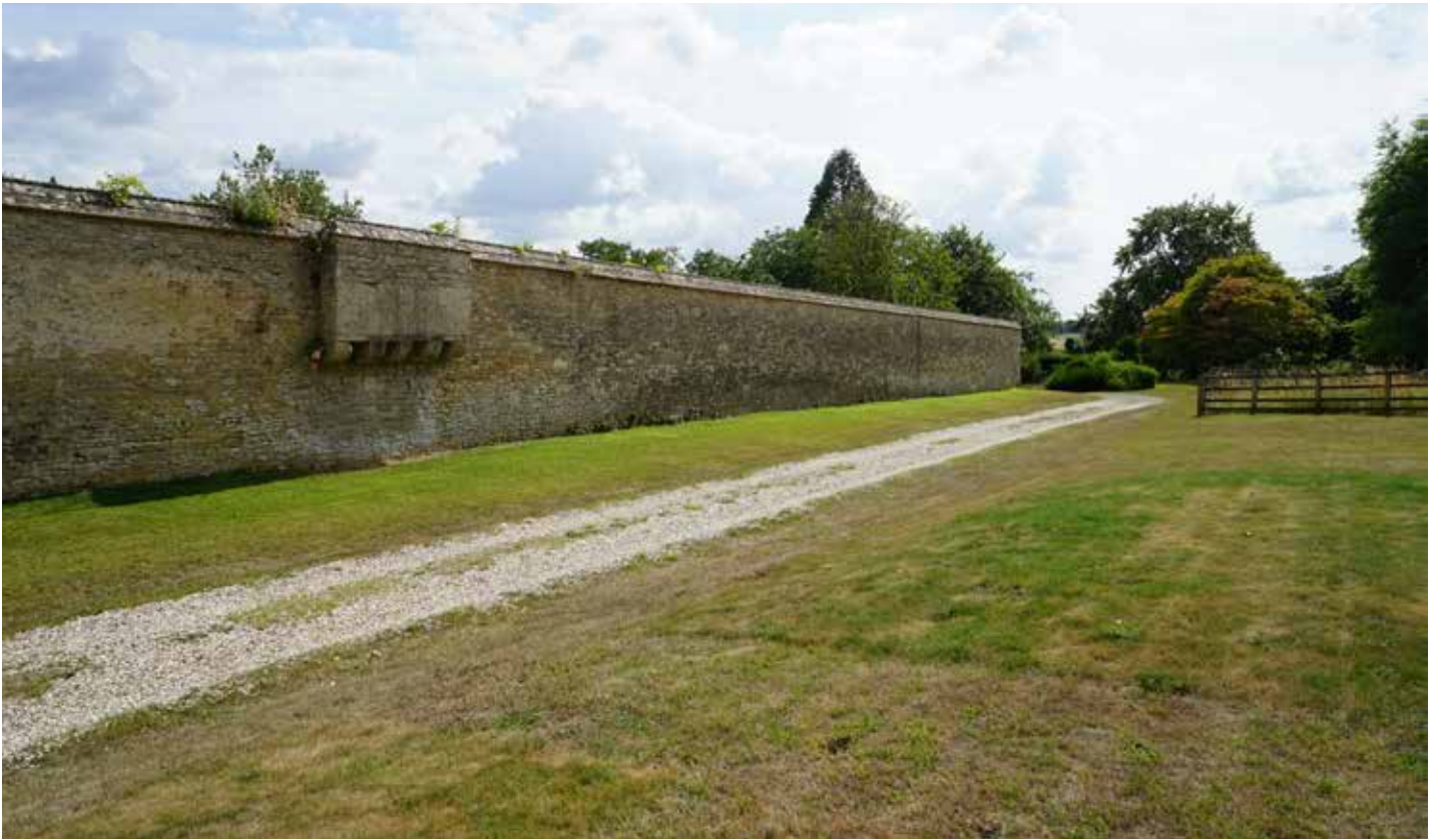
Enclosing wall with machicolations detail .
