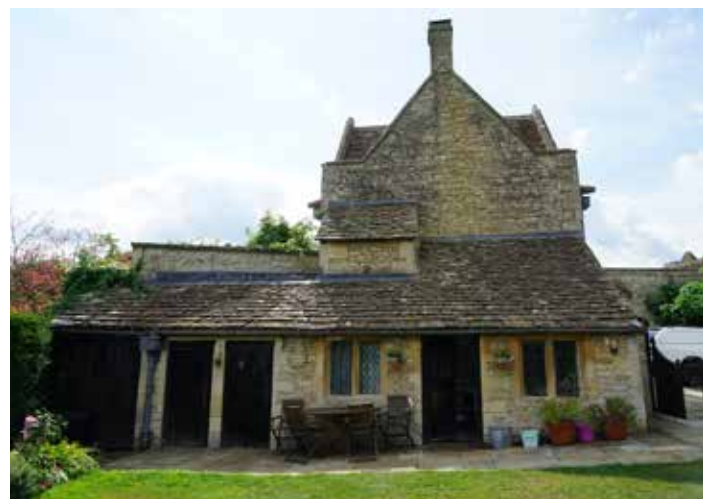
Dower House east elevation with single storey single pitched roof over kitchen and outhouses.
