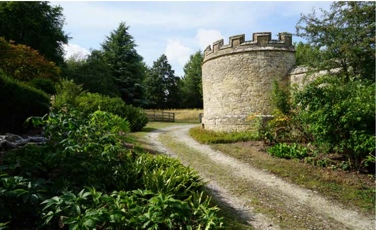
Castellated turret to north-west corner of the enclosing wall.
