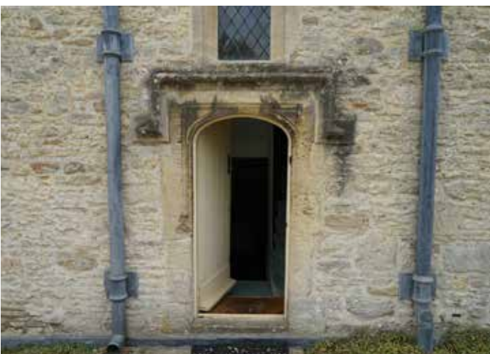
Central access door to rear (north) elevation with hood mould over arched door.
