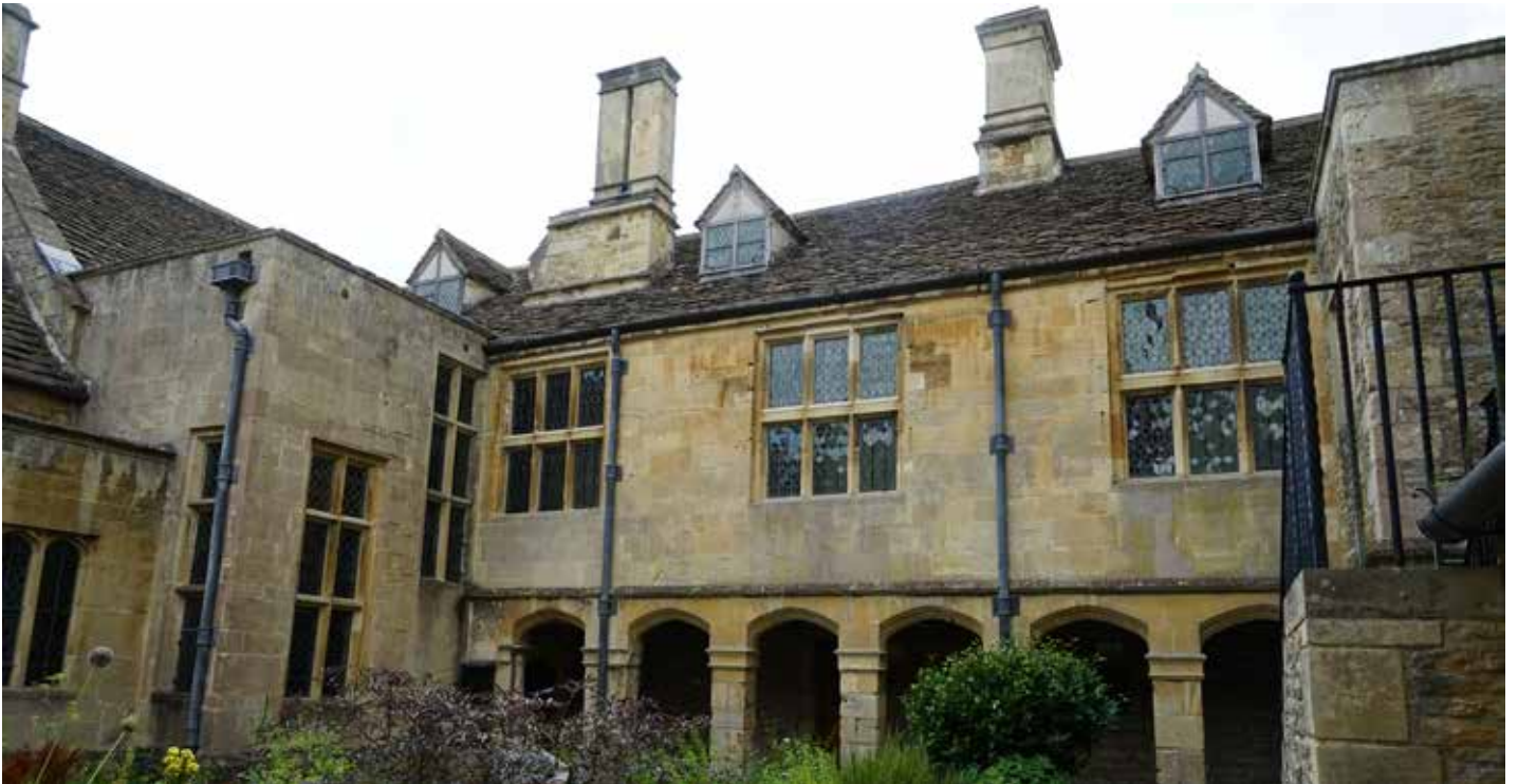
The south (left) and west (right) sides of inner central courtyard with original early and late 16th century windows.
