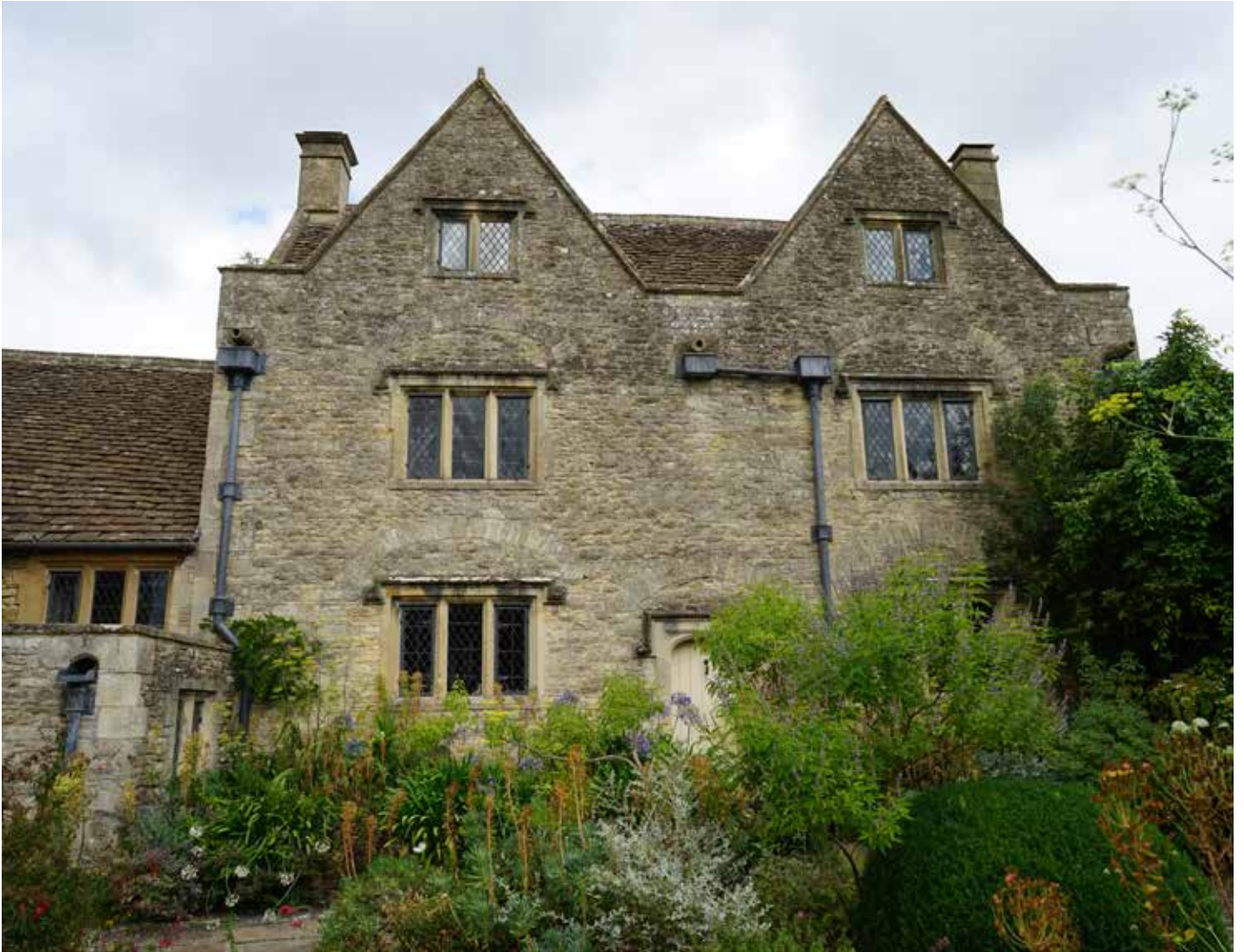
Dower House south elevation, with symmetrical gable front and relieving arches over the openings at the lower levels. Early 20th century service range attached to the left (west) side.
