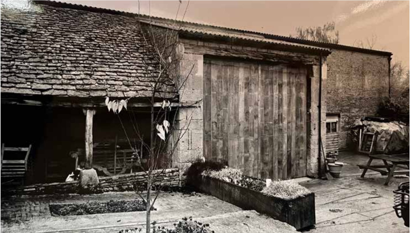
Barn to the west of the stable range 10 November 1994
