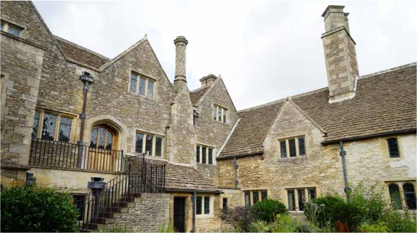
The north (left) side with steps leading down from first floor to garden level. The east (right) sides of inner central courtyard is noted as original up to the ridge stack.
