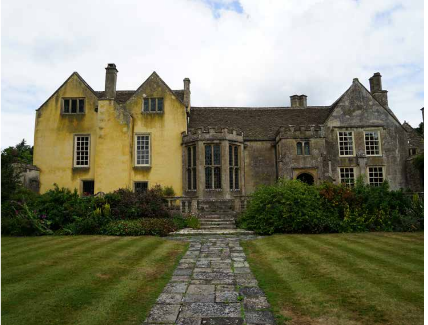
South elevation. The left hand range has been colour-washed in fairly recent years, making it appear quite different from the adjacent great hall range. The elevation appears more homogeneous in historic photographs.
