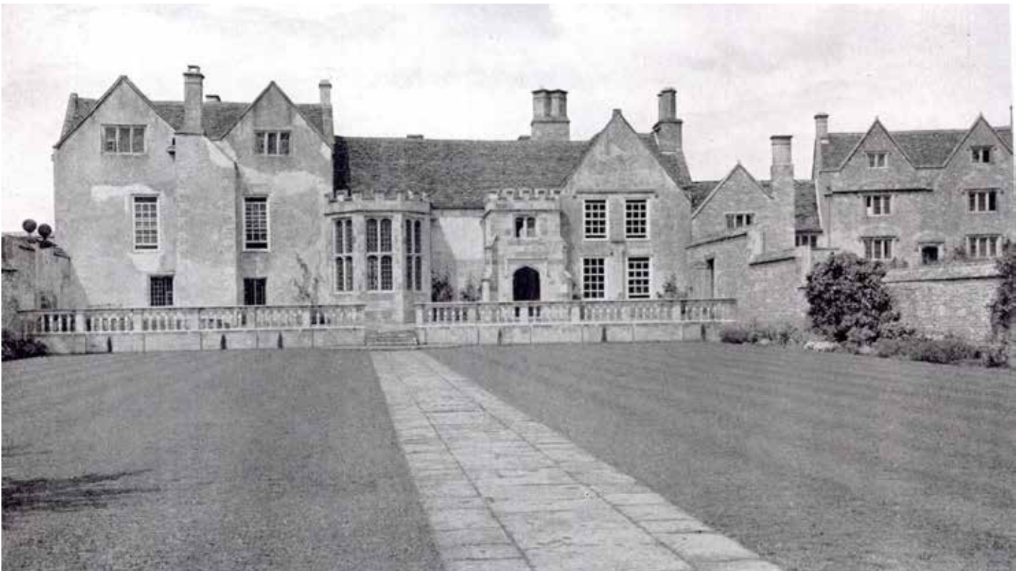
The south elevation with the oriel and porch the Dower House to the east with a new linking building
