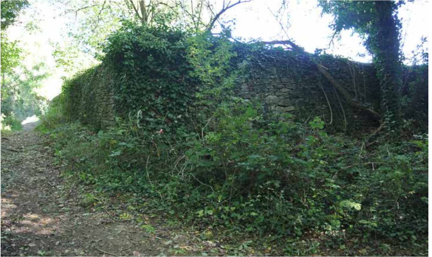
15a. Corner of drystone boundary wall at junction of footpath and bridleway.
