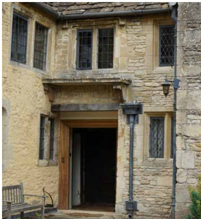
Open porch with long hood on carved 18th century brackets.
