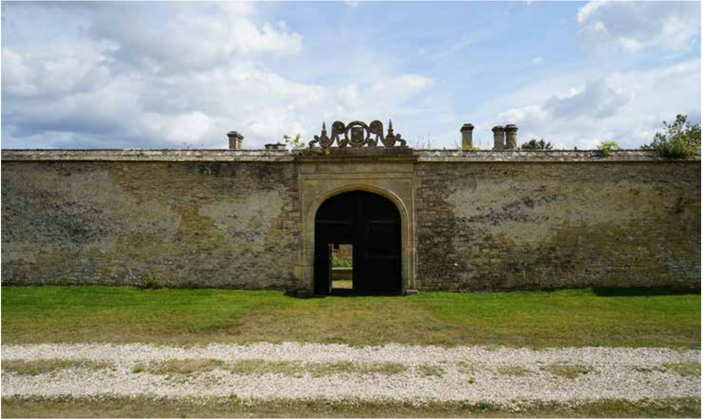
Enclosing wall with central four-centred arch gate.
