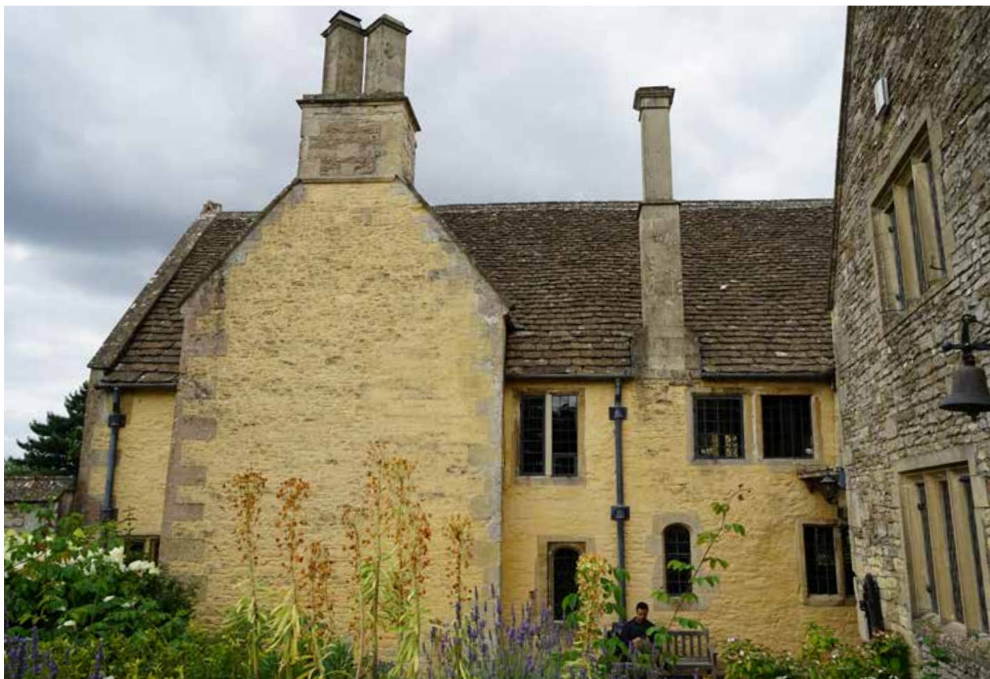
The east elevation of the main house front range, dominated by large wall-face stack. Entrance door to the right (canopy just seen).
