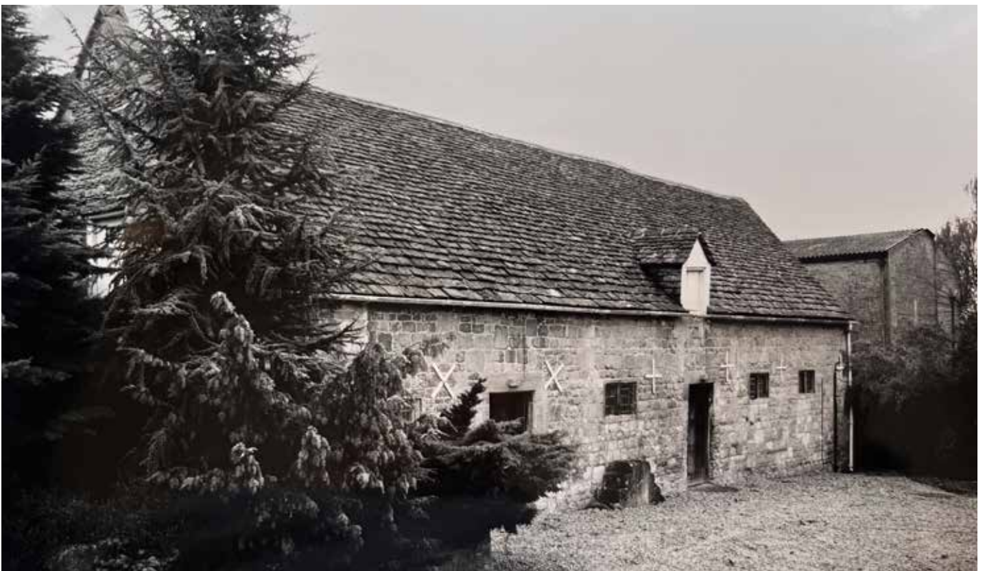
Stables viewed from the north 10 November 1994
