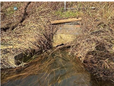
Figure 2-6: Culvert 1, Mason Arch Culvert
