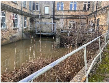
Figure 2-9: Sluices under building
