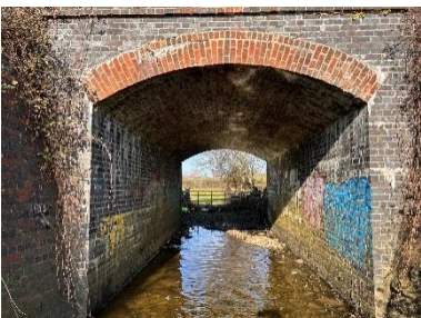
Figure 2-8: Culvert 2, Mason Arch Culvert
