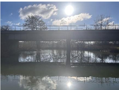
Figure 2-3: Railway Bridge Wessex Mainline
