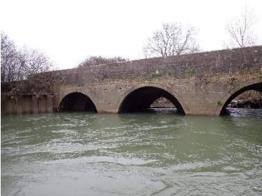
Figure 2-12: Road Arch Bridge on the River Avon
