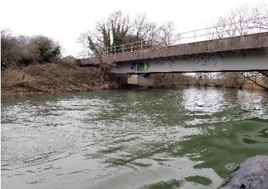
Figure 2-2: Railway Bridge Weymouth Line
