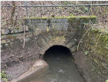
Figure 2-5: Culvert 0, Mason Arch Culvert
