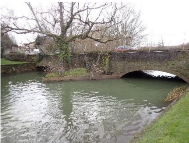
Figure 2-11: Weston Cut Bridge
