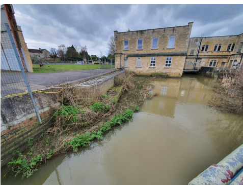
Figure 2.3: Weston Cut looking down-stream running under the Mill Building
