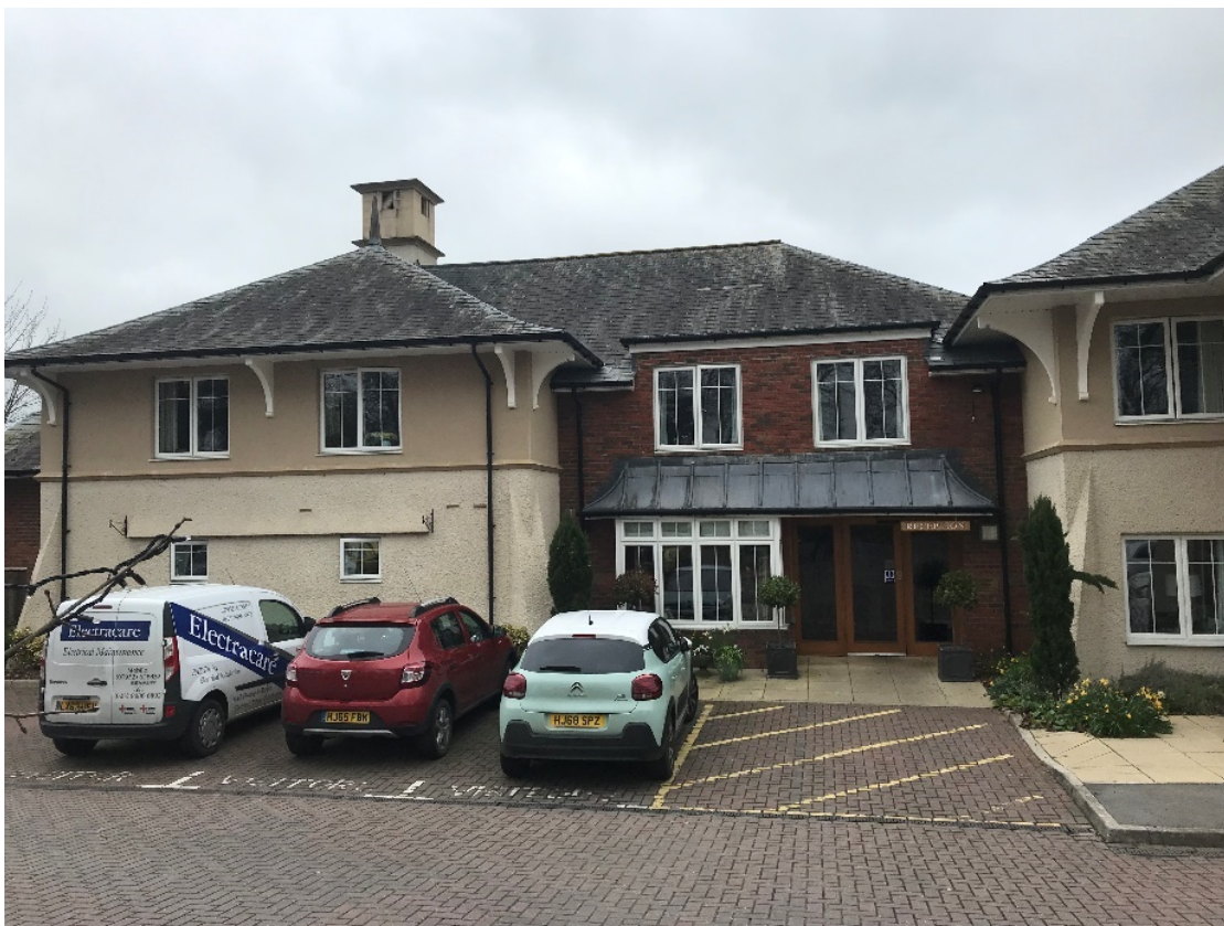
Photograph 7: B2; south-east wing, north-east aspect. View from north-east.
