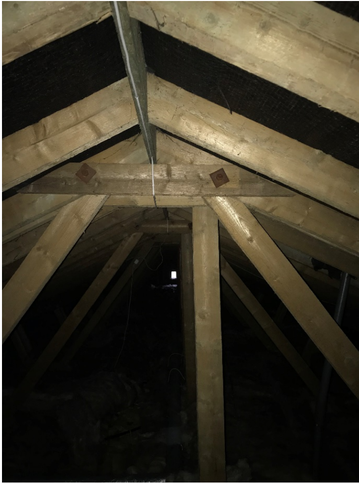
Photograph 6: B1; south-east wing loft void.
