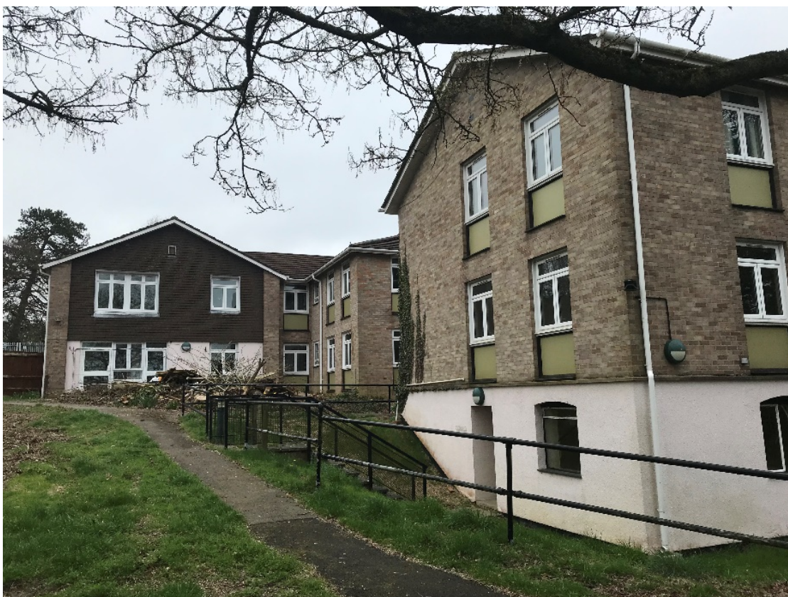
Photograph 1: B1; north and west wing; north-west aspect; view from the western site corner.
