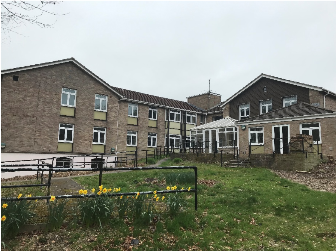
Photograph 3: B1; west and south-east wing; south aspect; view from the southern site corner.
