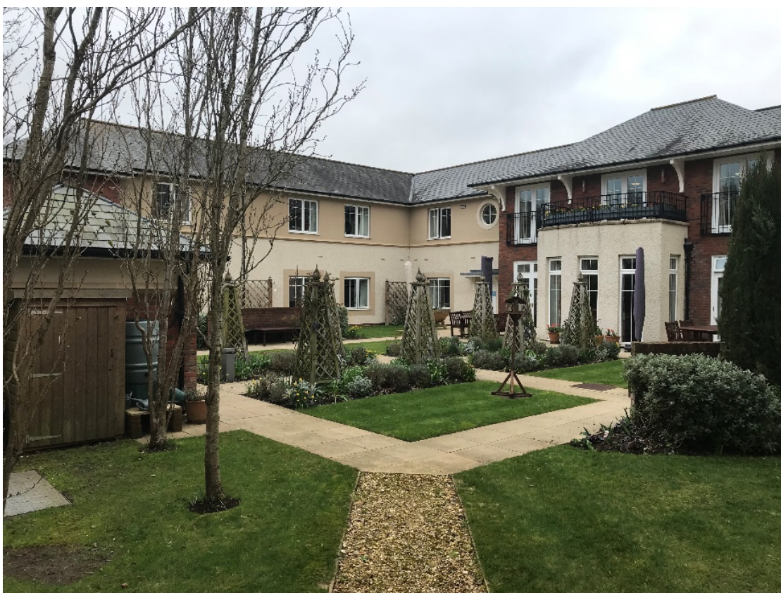
Photograph 8: B2; courtyard between south-west, north, and south-east wing. View from south.
