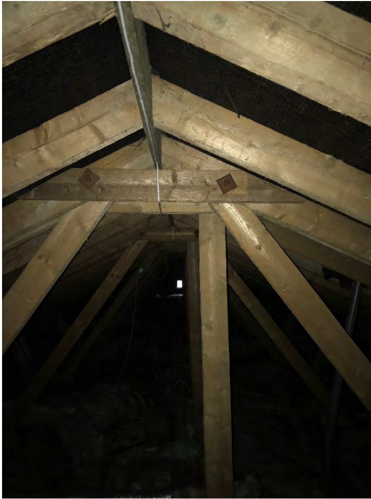
Photograph 6: B1; south-east wing loft void.
