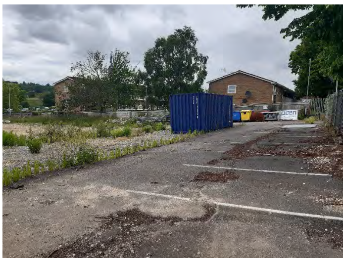
Photograph 1: Tarmac hardstanding at site entrance.
