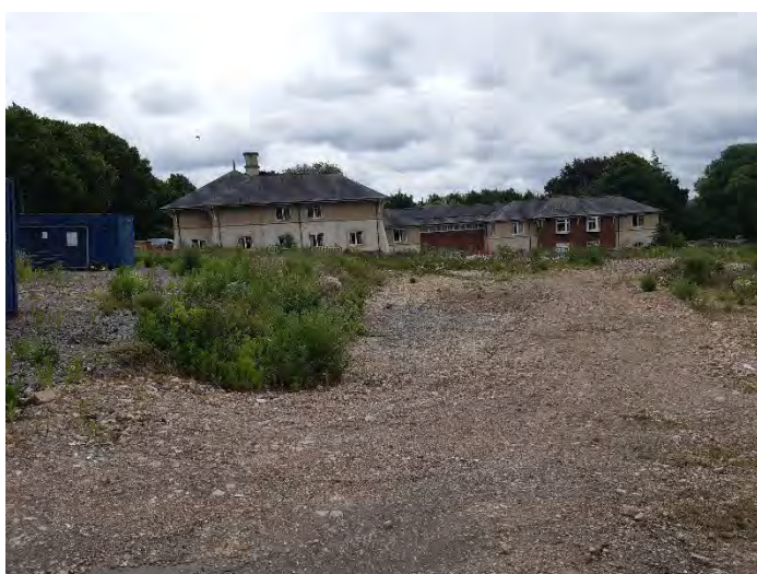
Photograph 3: Large areas of bare ground created from rubble following the demolition of Stratford Court. The adjacent Braemar Lodge is shown in the background.
