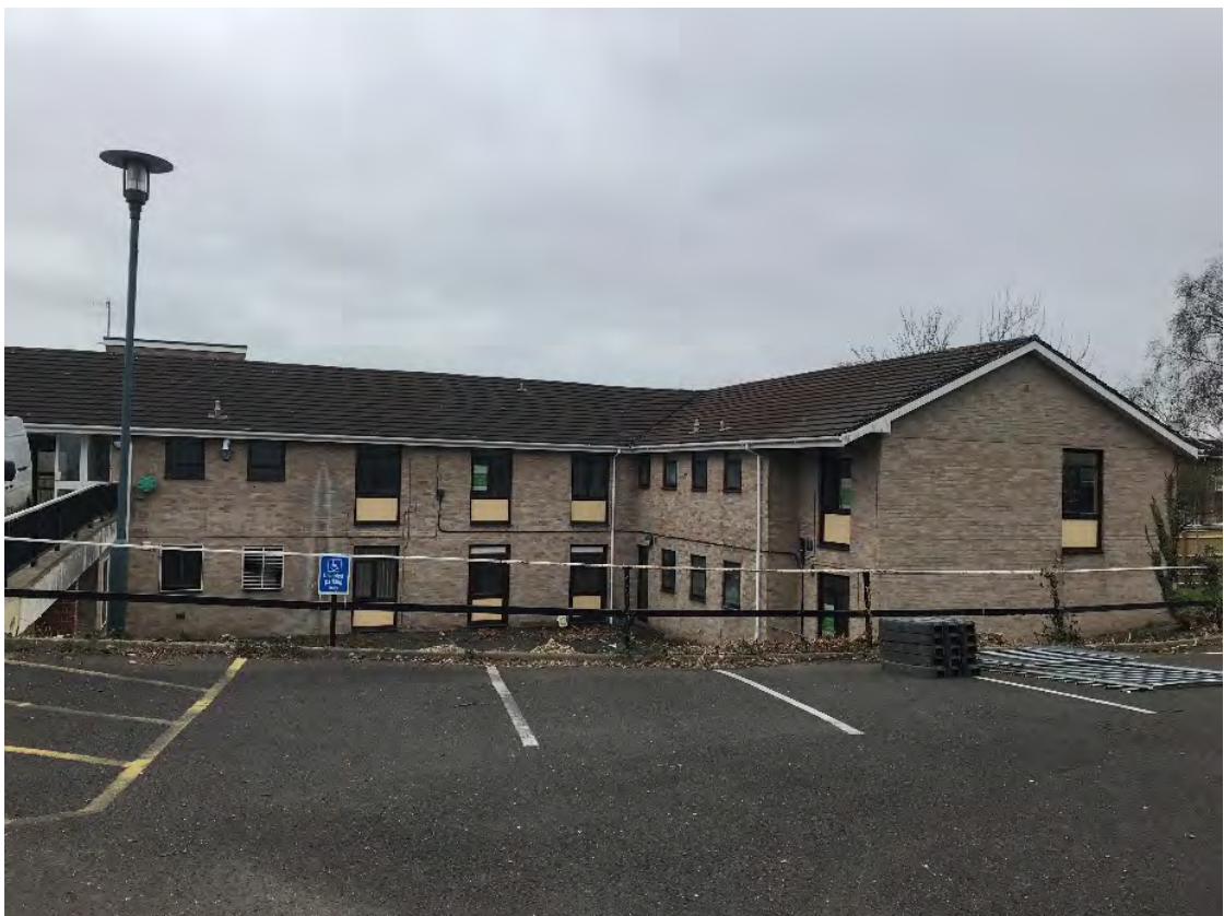
Photograph 2: B1; north wing; north-east aspect; view from the northern site corner.
