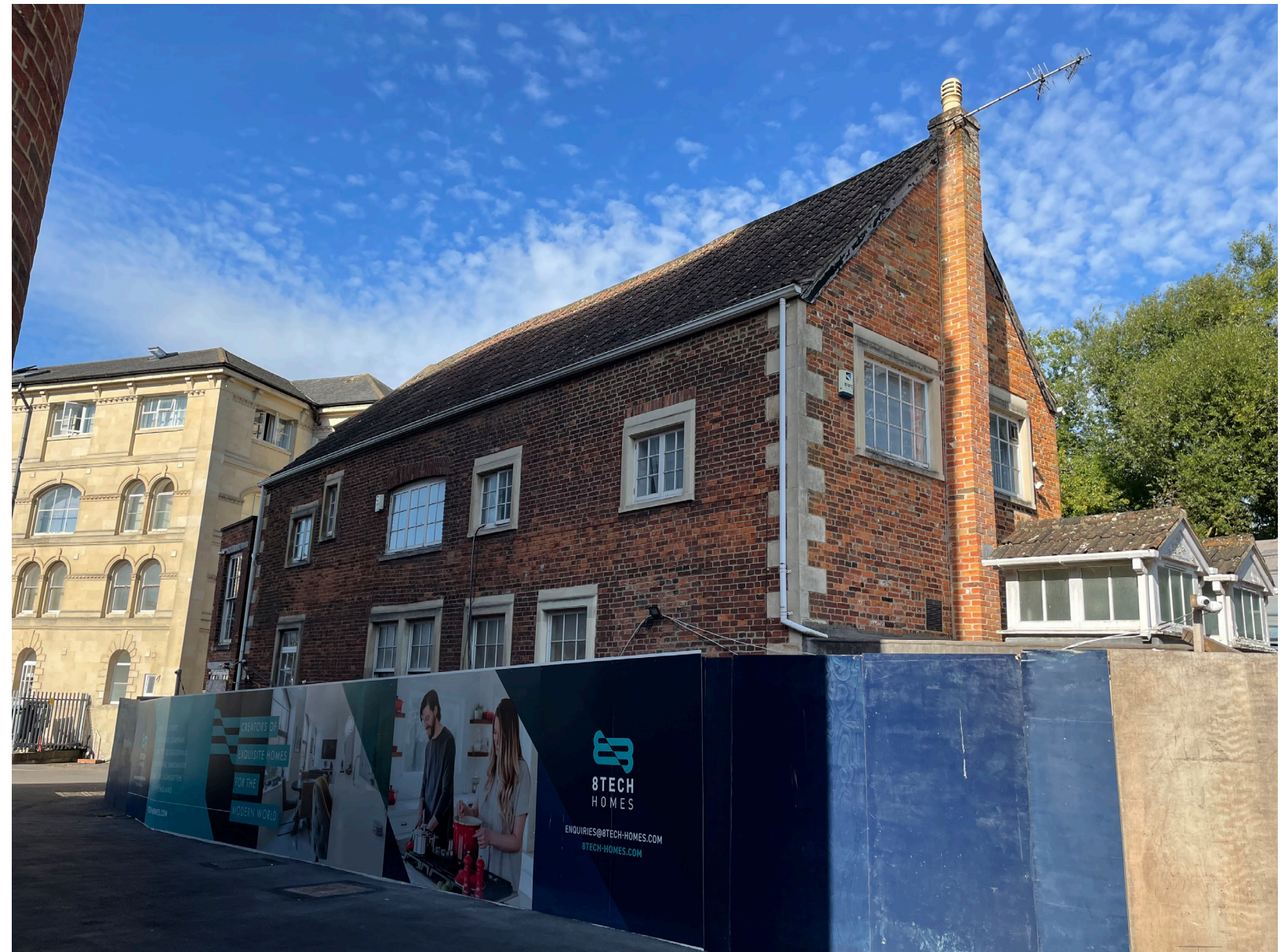
Above: Mill House, as Existing Photograph: October 2023
