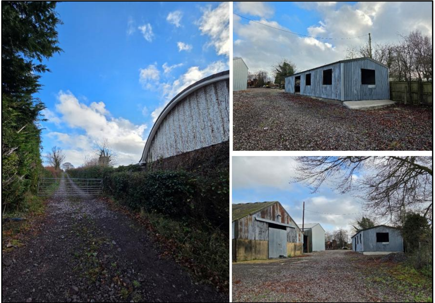
PHOTO 1 – Site Photos of Site Access & Existing Building
