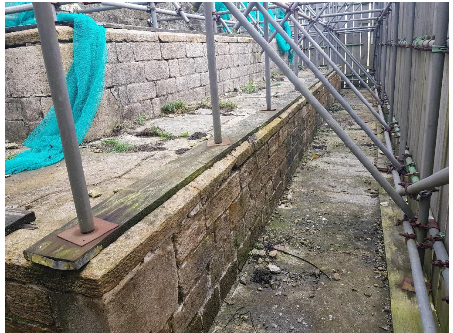
Figure 4 View of temporary scaffold structure from within the timber hoarding
