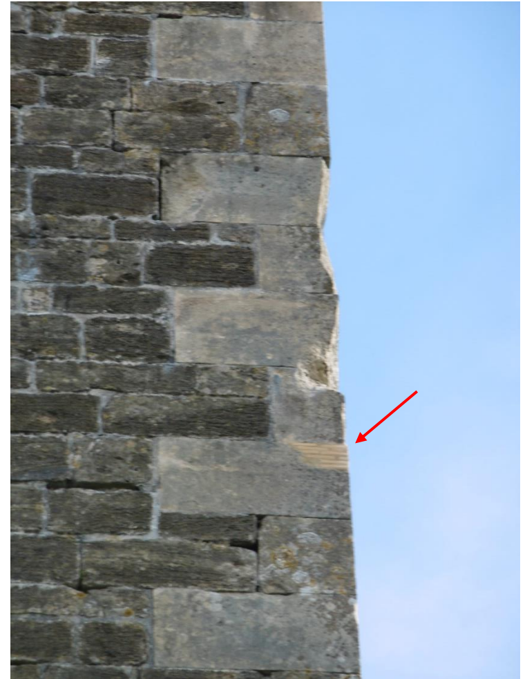
Figure 10 Sample tile repair to a partially-decayed quoin at the south corner of the main shaft
