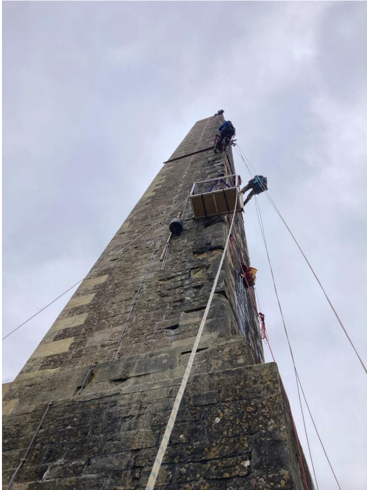
Figure 7 Installation of new trial quoin stones to the west corner of the monument using purpose-made working platform (2024)
