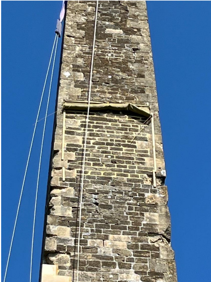
Figure 9 Re-pointing trials to south-west face of the main shaft (with temporary protective sheeting rolled up at the head)
