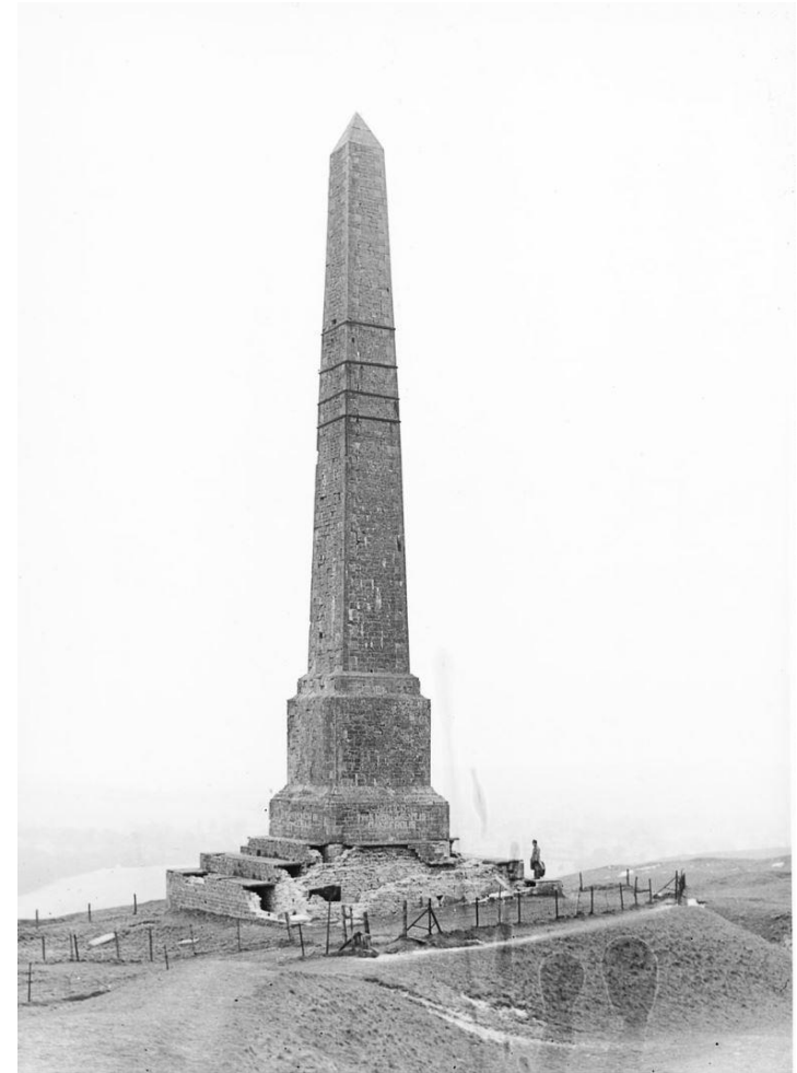
Figure 6 View of monument in the mid-20 th century with iron bands around the main shaft
