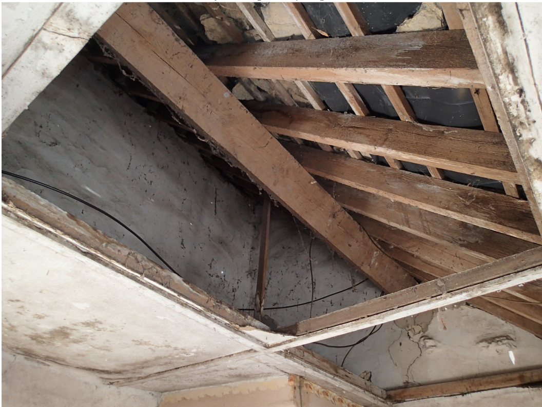
House – loft (temporary repair visible)
