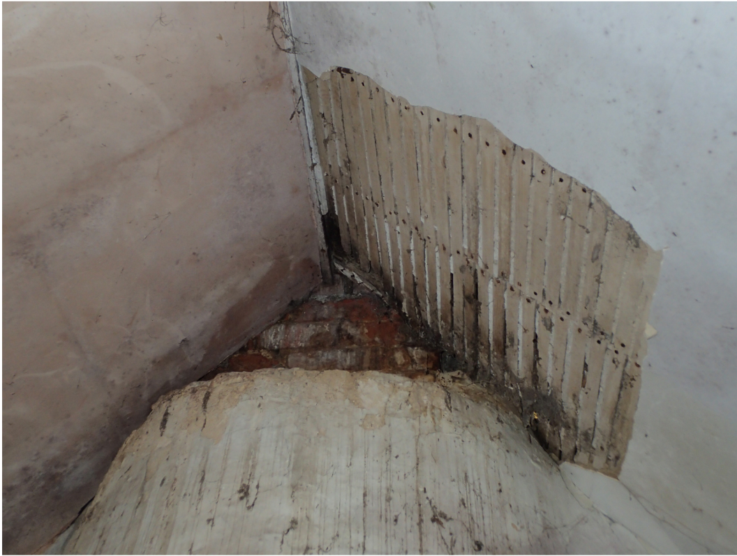
House – example room in roof space
