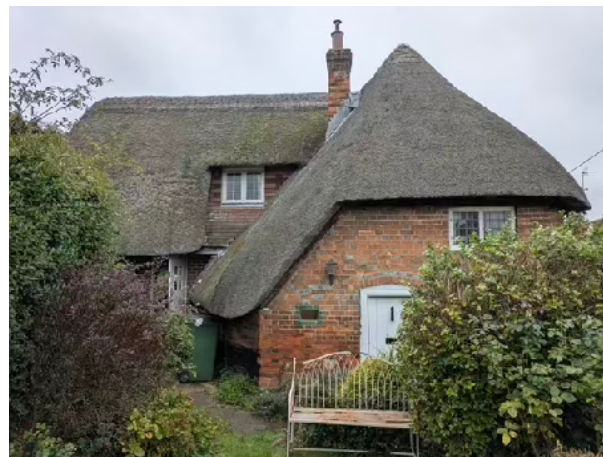
2. The southern elevation cobbler workshop extension and rear extension
