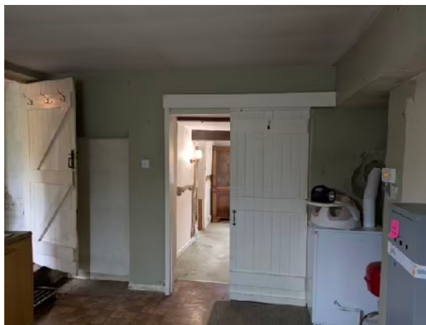
11. Kitchen doorway and blocked cross passage door to left
