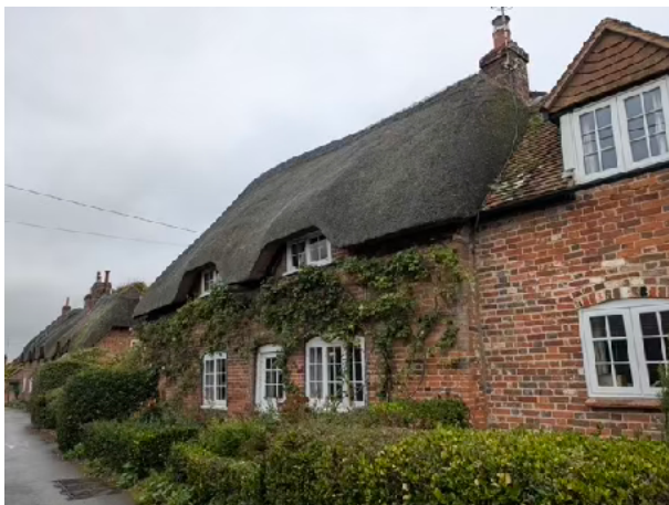
1. No.35 Farm Lane, Cobbler's Cottage
