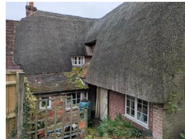
3. Rear courtyard and extension
