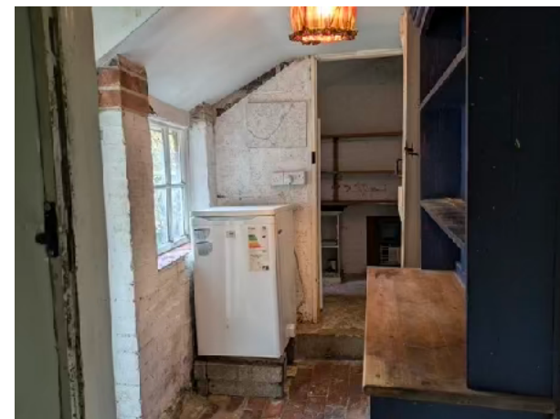
12. Rear utility; blockwork and new brick walls
