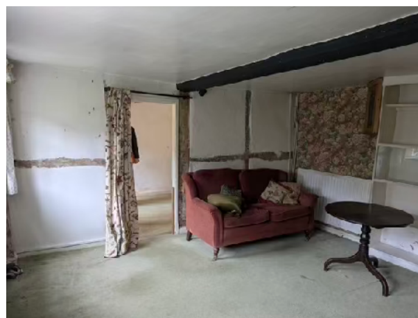
5. Main reception box framing
