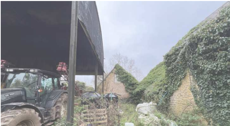
Fig.38 View of Existing
