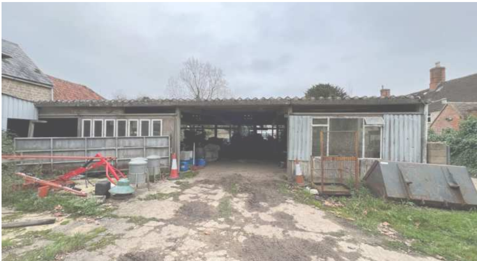
Fig.33 View of Existing
