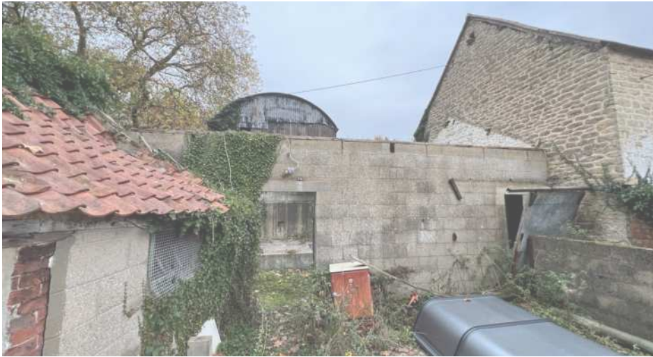
Fig.30 View of Existing
