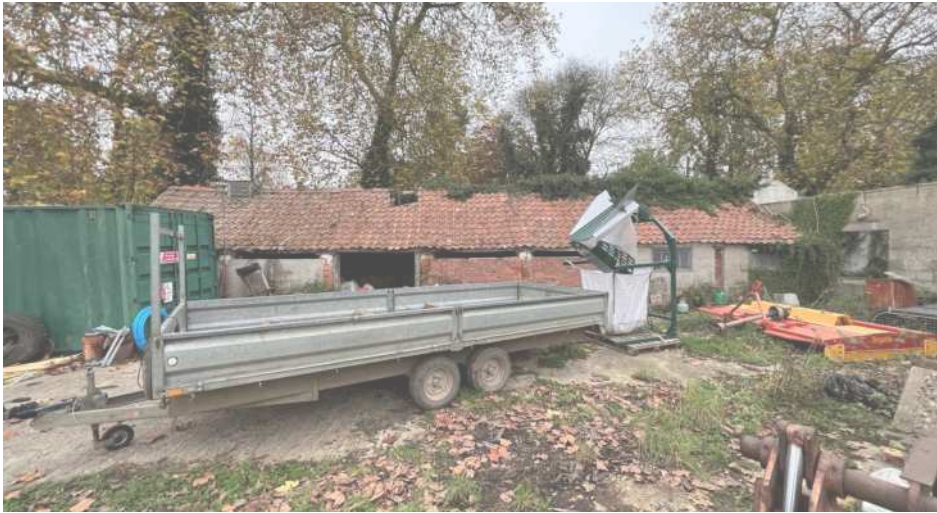
Fig.26 View of Existing
