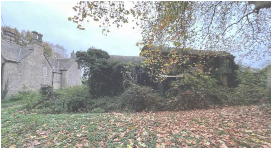
Fig.43 View of Existing
