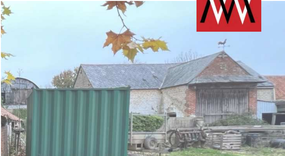
Fig.09 View of Existing
