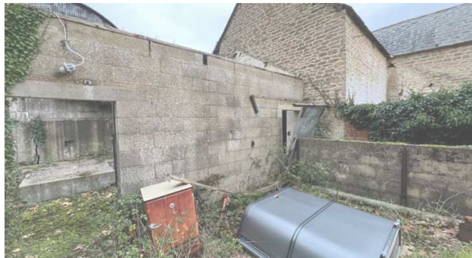
Fig.14 View of Existing
