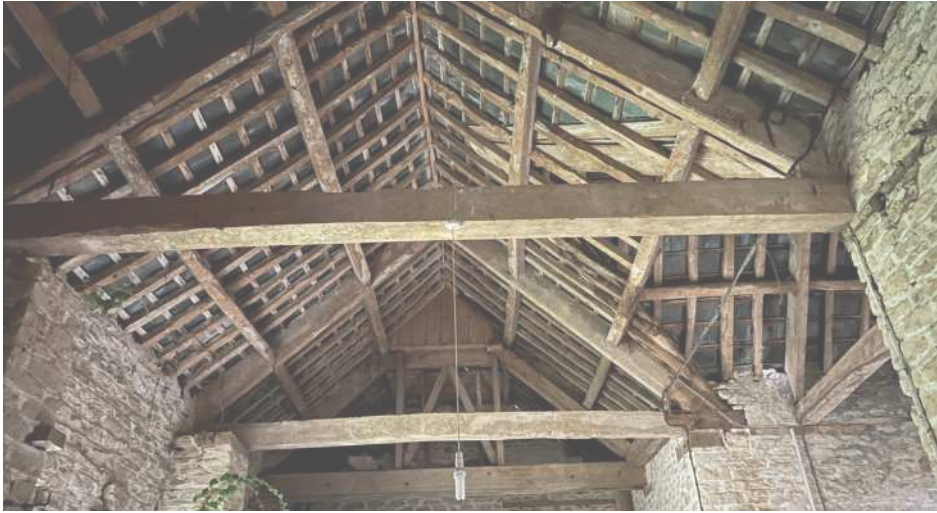
Fig.11 View of Existing
