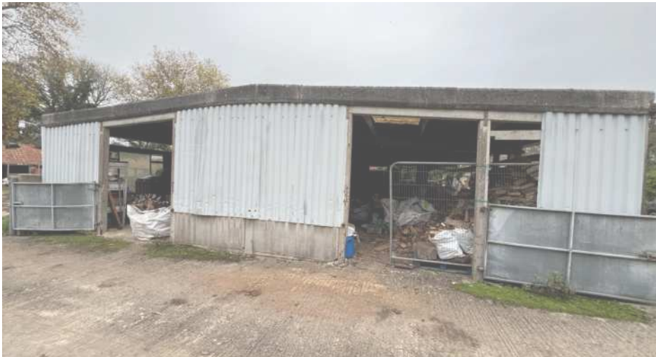
Fig.32 View of Existing
