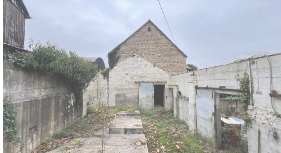
Fig.12 View of Existing
