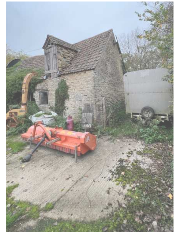
Fig.24 View of Existing
