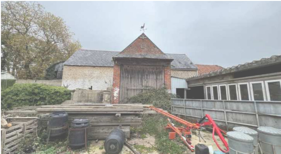
Fig.05 View of Existing
