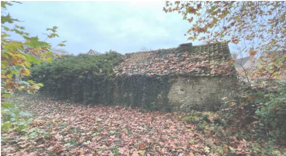
Fig.25 View of Existing
