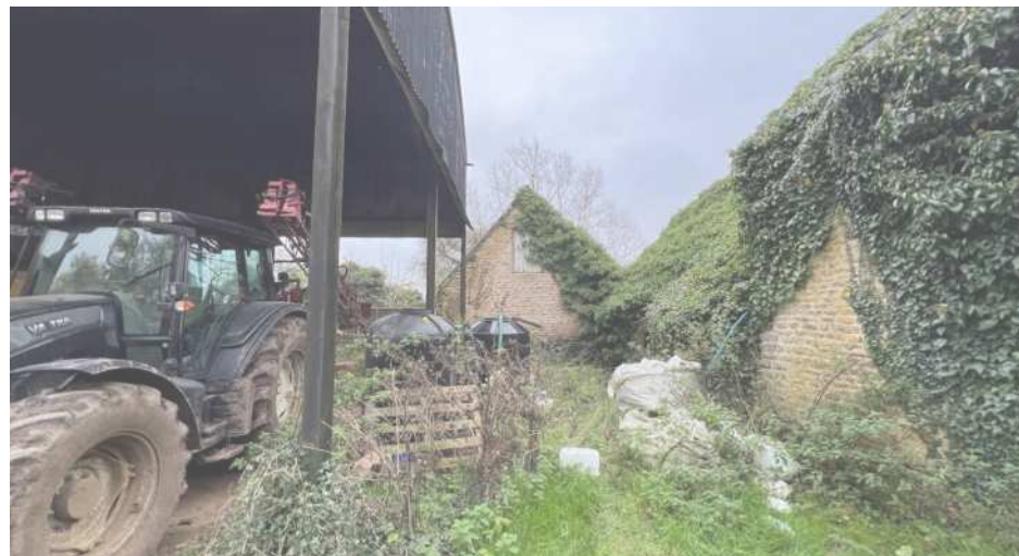
Fig.21 View of Existing
