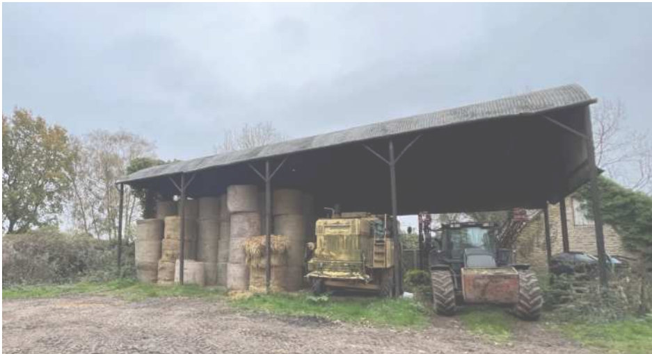
Fig.37 View of Existing
