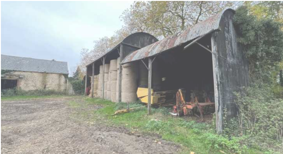
Fig.42 View of Existing
