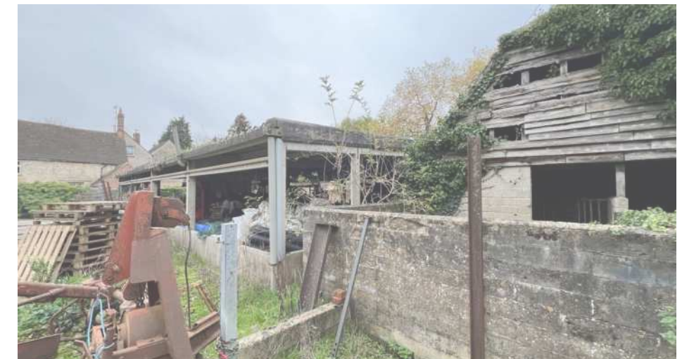
Fig.18 View of Existing
