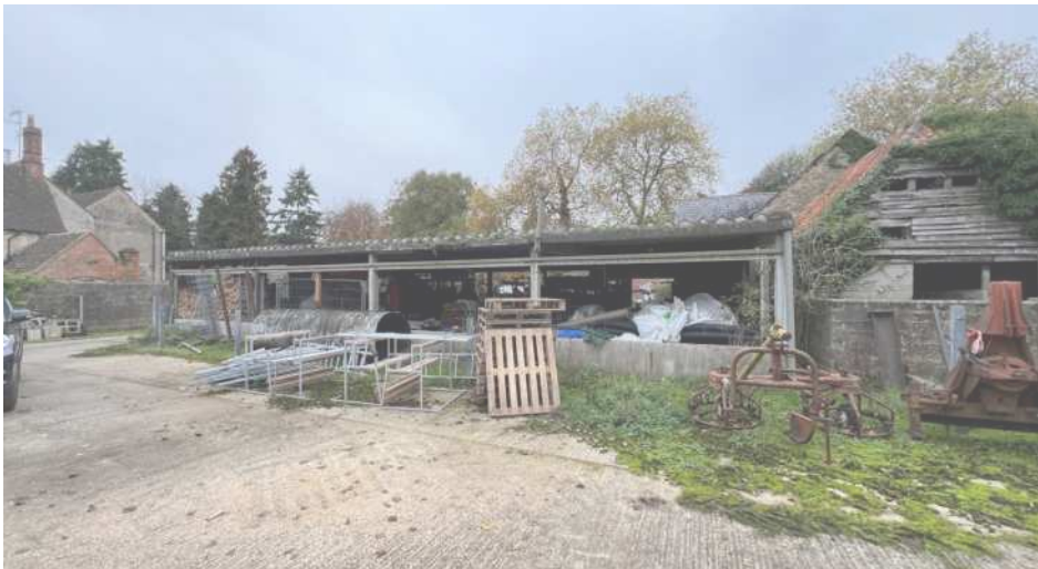
Fig.32 View of Existing
