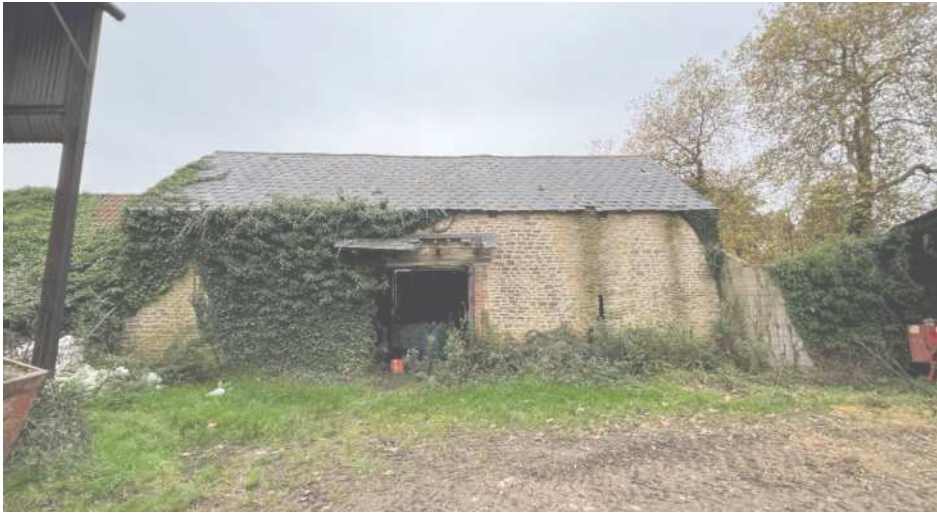
Fig.06 View of Existing
