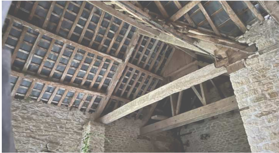
Fig.10 View of Existing
