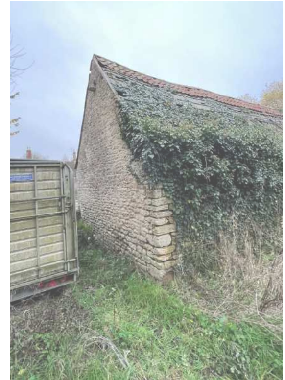
Fig.23 View of Existing
