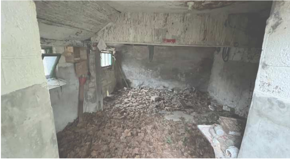
Fig.27View of Existing
