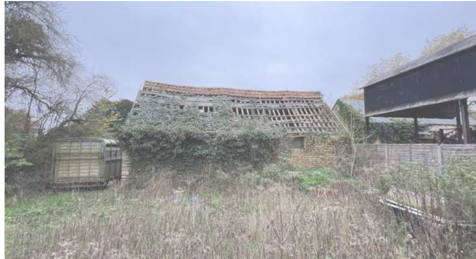
Fig.20 View of Existing
