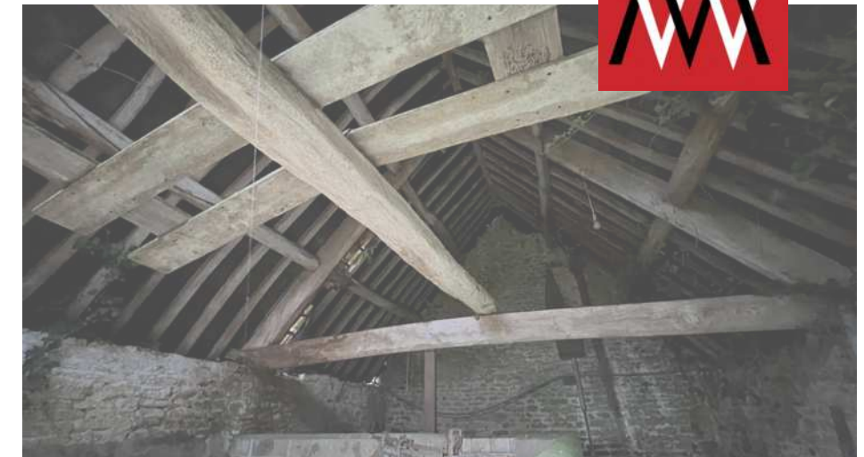
Fig.16 View of Existing
