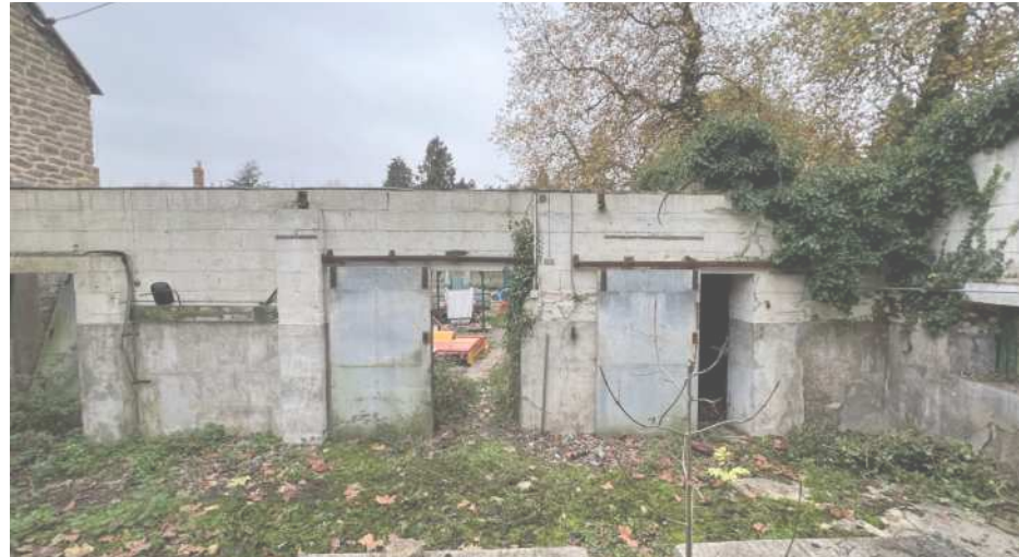
Fig.13 View of Existing
