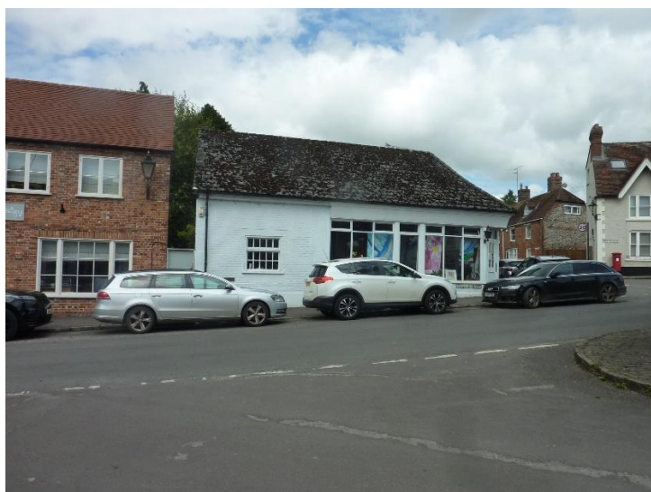
Figure 3: View of part of the front elevation from High Street
