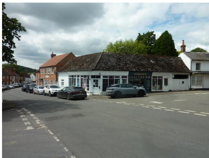
Figure 4: View of front elevation from within The Square
