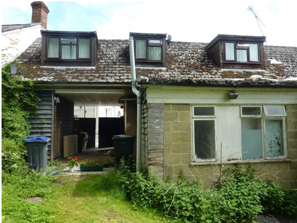
Figure 9: Dormer windows on the attached neighbouring property.
