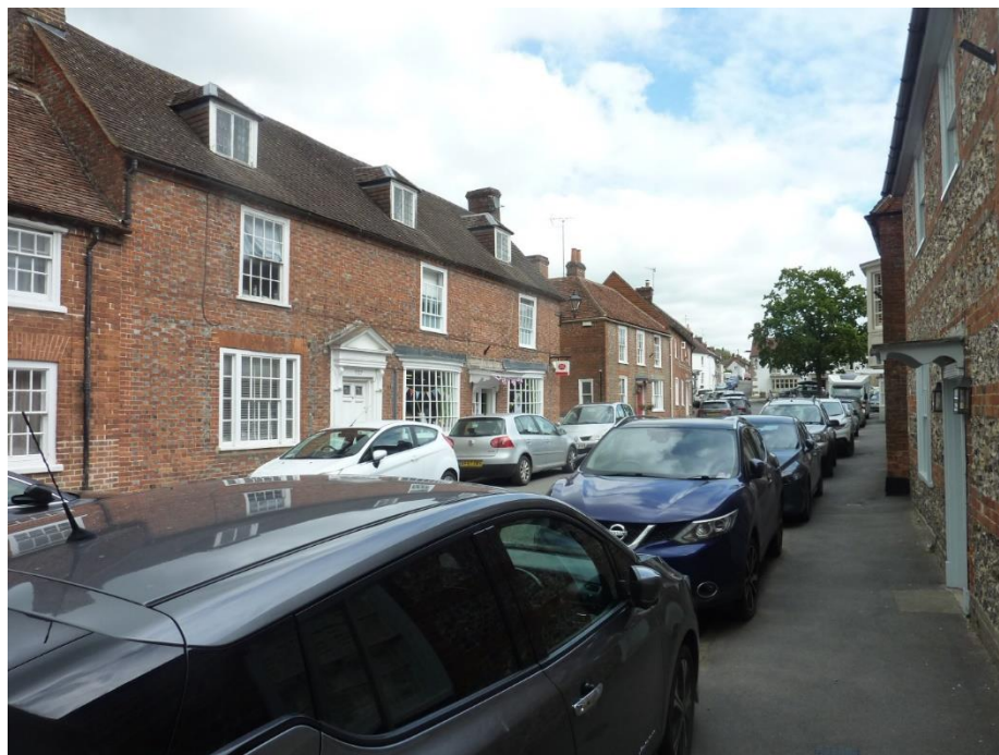
Figure 8: Dormer windows on a front facing roofslope at High Street.
